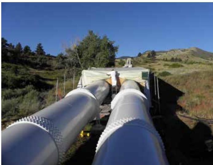
Flatiron Penstock Coating Project - CO
