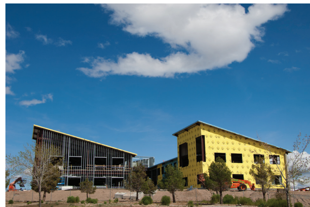
The Green Building under construction in Boulder City, Nev.
