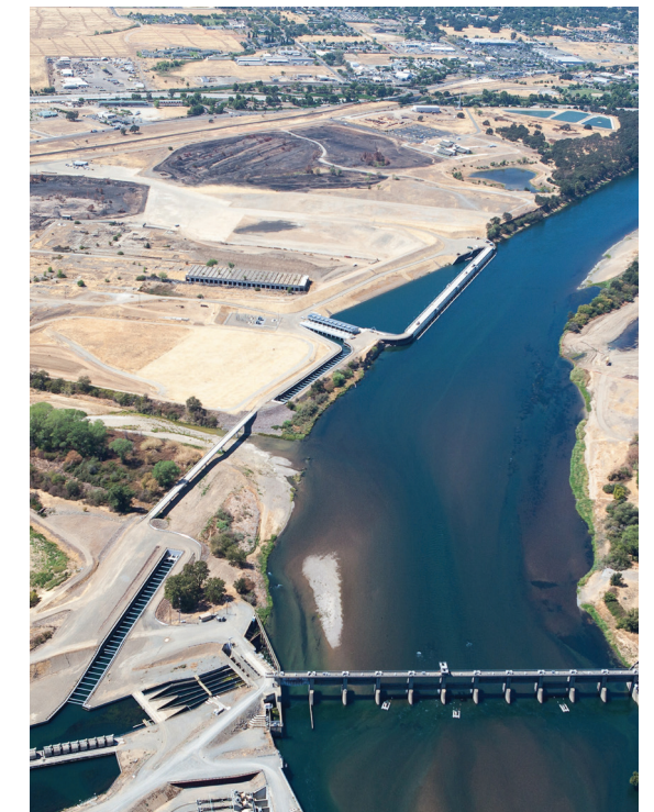
Red Bluff Fish Passage Project
