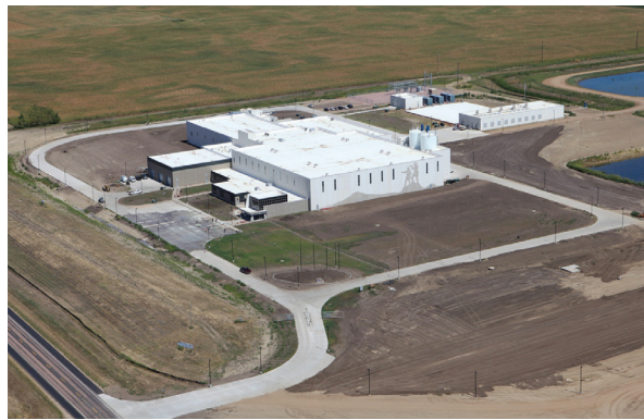
Lewis and Clark Regional Water System
