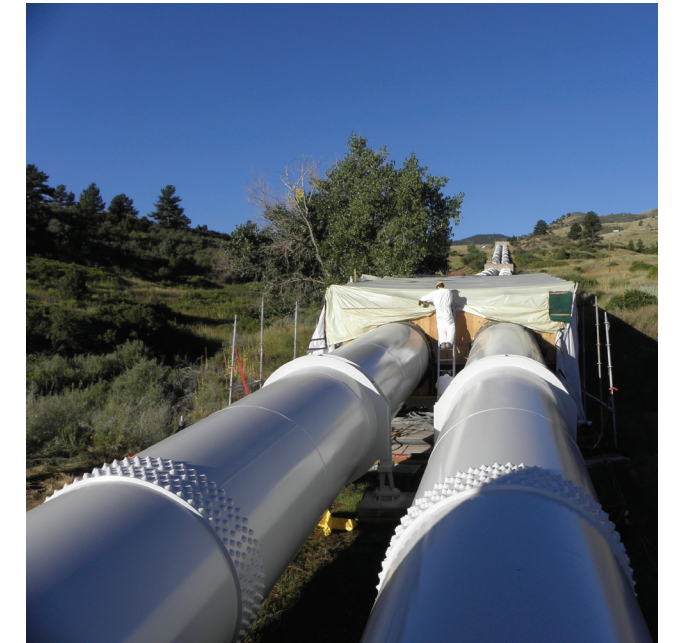
Flatiron Penstock Coating
