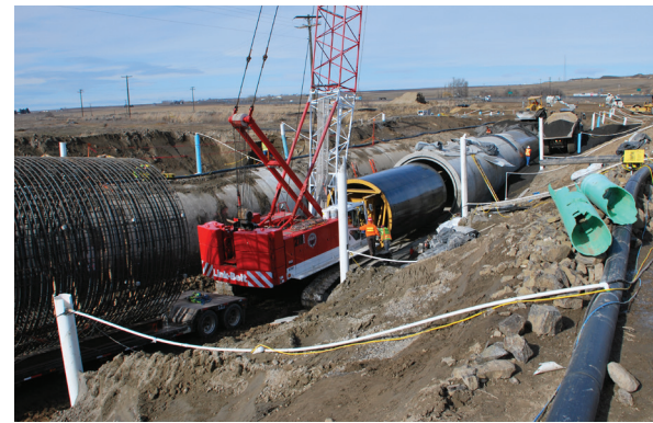
Weber Siphon being constructed.
