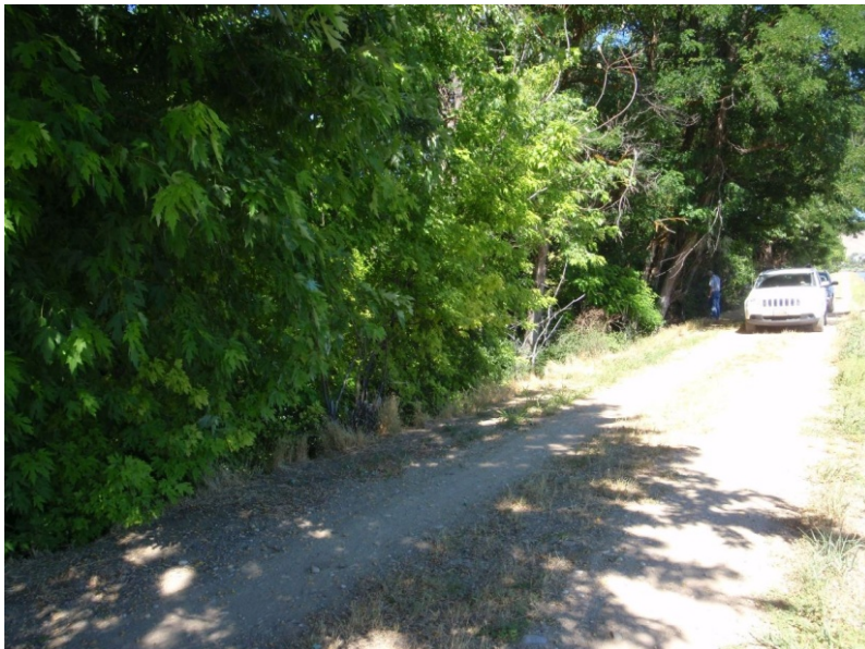
Figure 14. Large and dense trees growing on the outside slope of the canal embankment.
