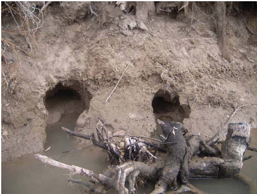
Figure 12. Large and small diameter animal burrows on the inside of the canal prism.
