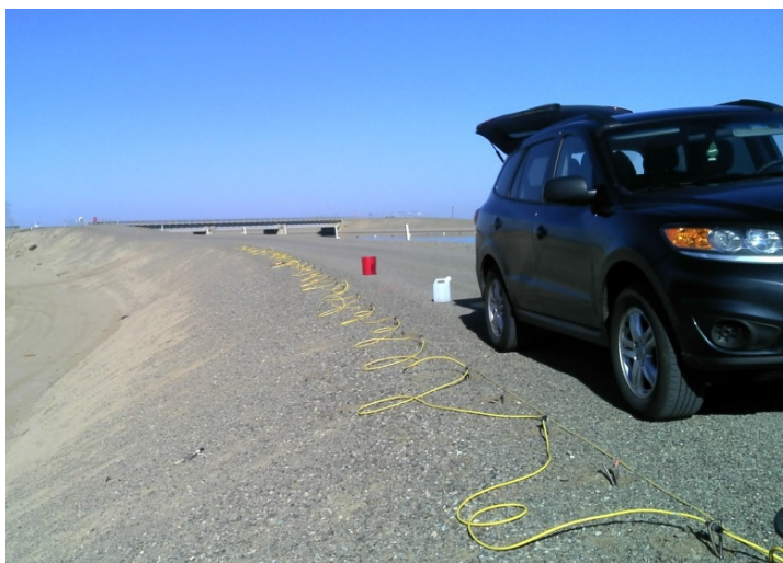
Figure 8. Collecting geophysical data on a suspected seepage area in a canal embankment.
