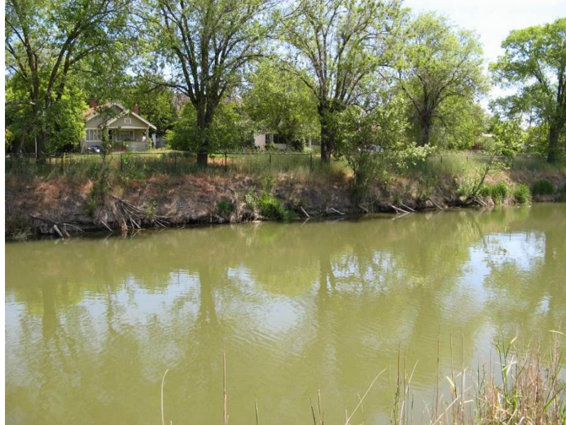
Figure 13. Trees growing on inside of canal prism; note roots.
