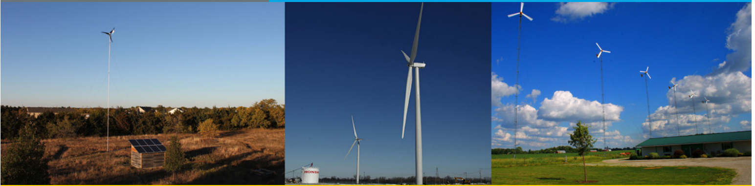
The distributed wind market includes wind turbines and projects of many sizes, such as a Pika T701 1.80-kW wind turbine paired with a 2-kW solar array in Kansas, two GE 1.7-MW wind turbines at a Honda transmission plant in Ohio, and six Bergey Excel-S 10-kW wind turbines in Ohio. Photos from left to right: from Kelsey Kaufman; from Honda.com; from Mark Spears.
