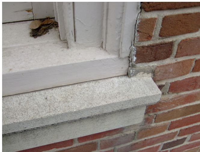
Figure 10. Wood window sill on top of masonry sill
