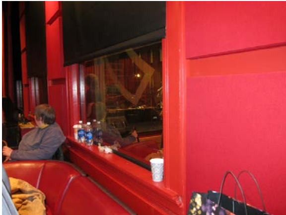
Figure 28. Interior storm window on double-hung original window
