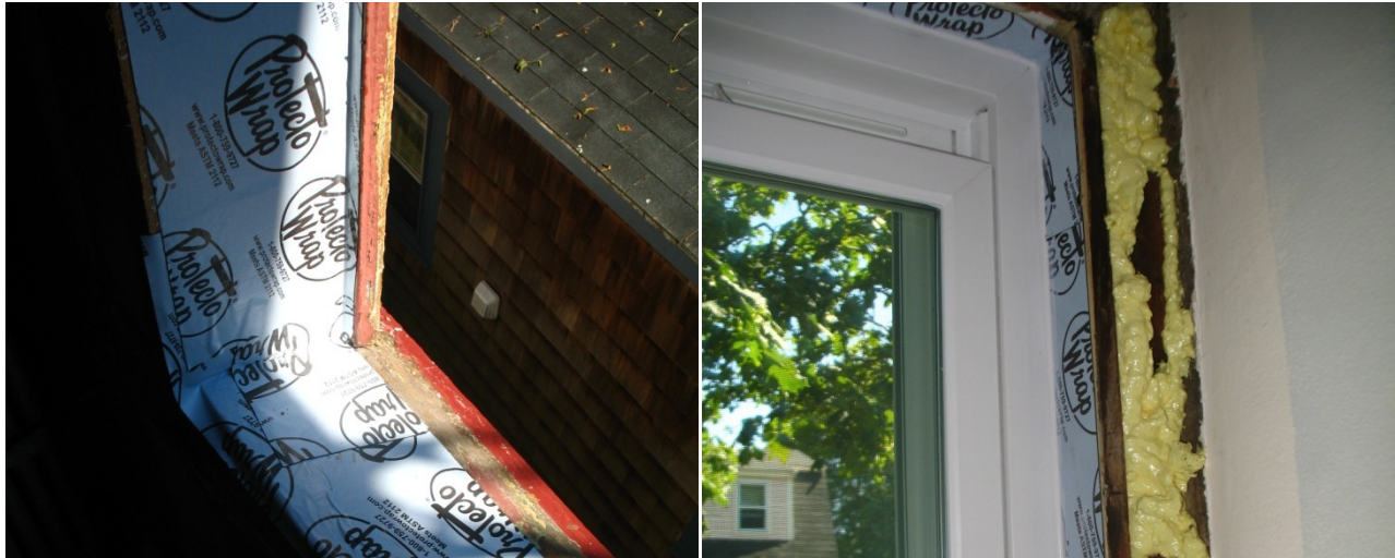
Figure 44. Examples of membrane installation in a wood window frame
