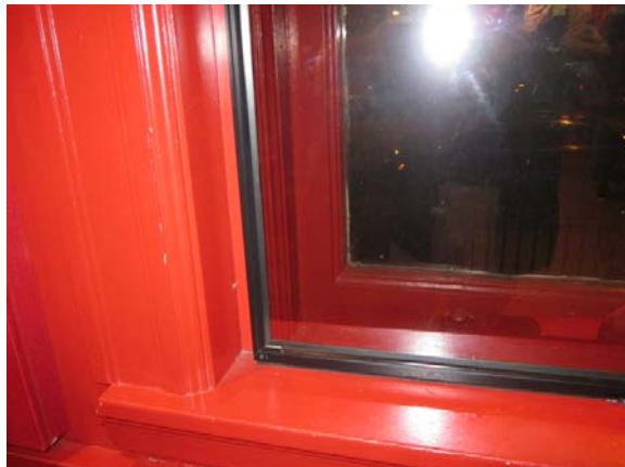
Figure 27. Interior storm window on double-hung original window
