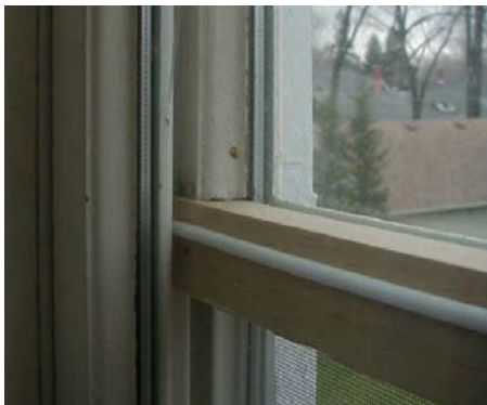
Figure 30. Window sash modification
