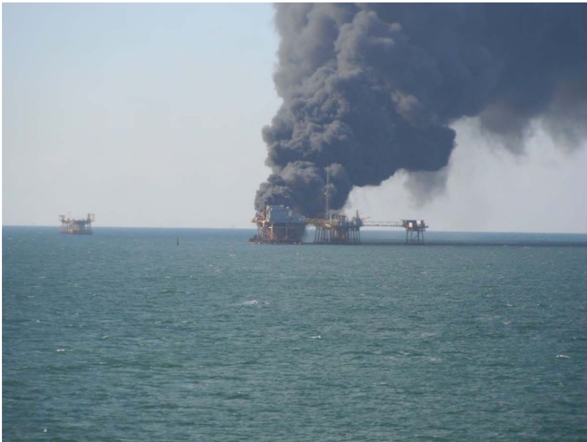
Figure 1 – WD 32 E platform after explosion
