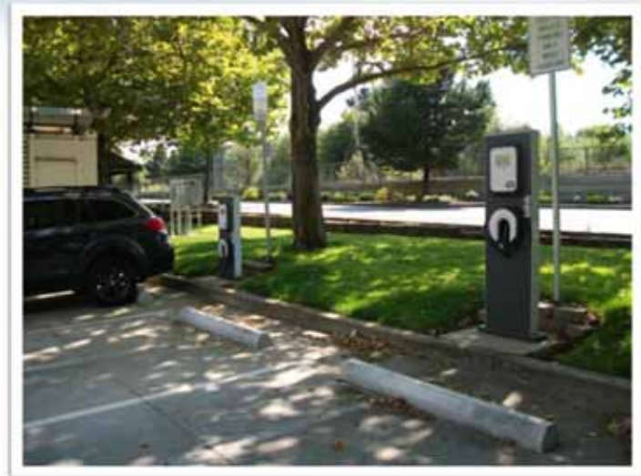
Pedestal EVSE installed on concrete pad, with underground boring for conduit
