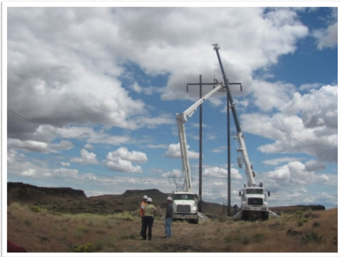
Figure 2-4. Removal of an Existing H-Frame Wood-Pole Structure
