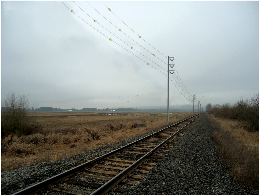
Figure 3-21. Viewpoint 3 - Proposed View of Structures SA1:12/3 to 12/2, with Bird Diverters, Looking North
