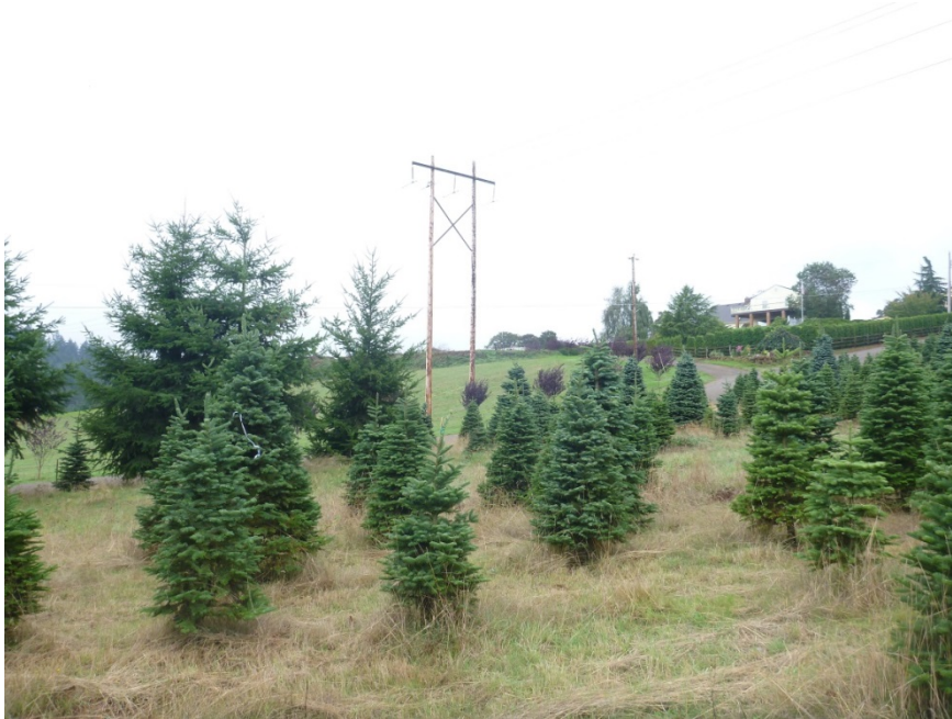
Figure 3-8. Transmission Line at Tree Farm, Looking at Structure SA1:6/8
