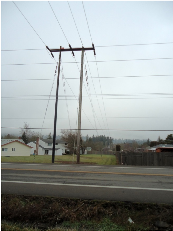
Figure 3-24. Viewpoint 5 - Current View of Structure SA1:21/8, Looking South
