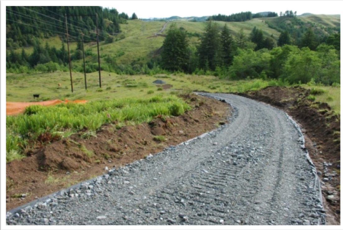
Figure 2-8. Improved Access Road
