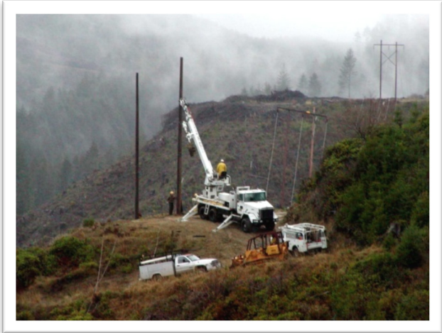
Figure 2-6. Installation of an H-Frame Wood-Pole Structure
