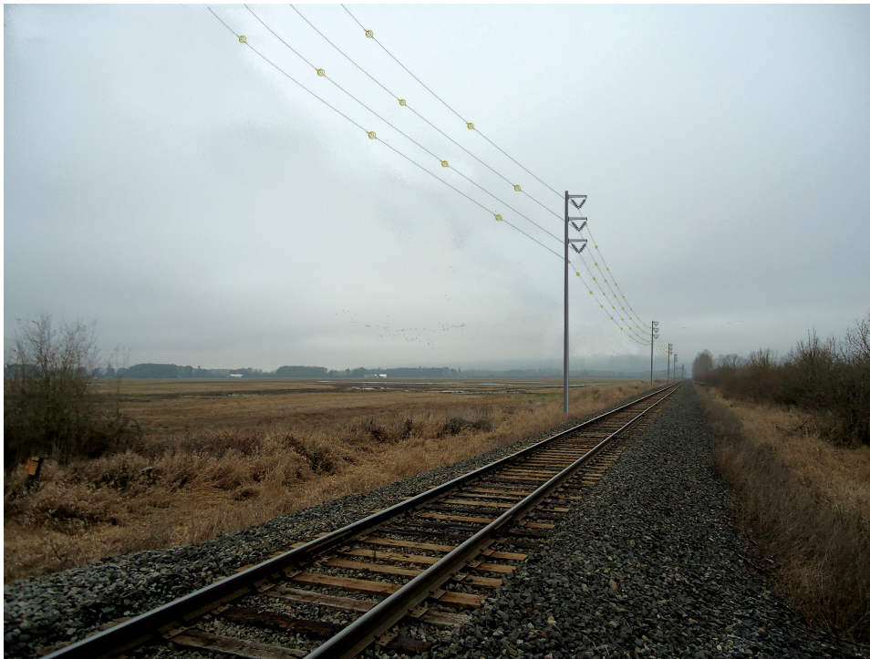
Figure 3b. Simulation of Proposed Steel Monopole Structures at SA1:12/3, with Bird Diverters and Conductors , Looking North
