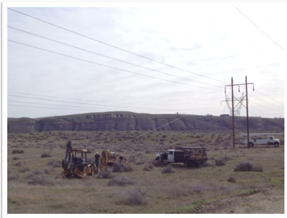
Figure 2-7. Conductor Tensioning after Conductor Installation
