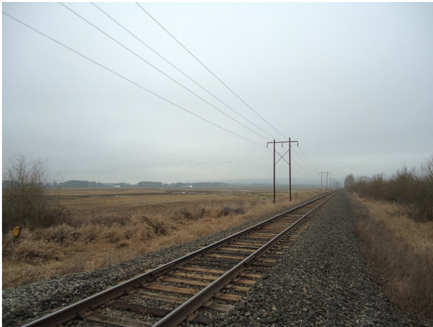
Figure 3-20. Viewpoint 3 - Existing View of Structures SA1:12/3 to 12/2, Looking North
