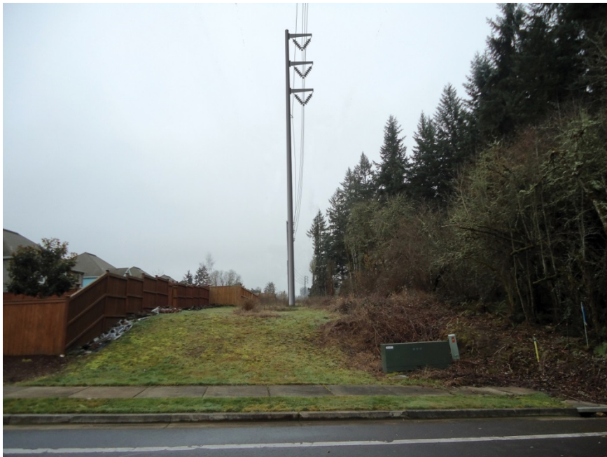
Figure 3-17. Viewpoint 1 - Proposed View of Structure SA1:21/2, Looking South
