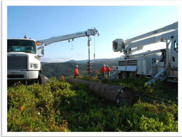
Figure 2-5. Auguring Holes for a Wood-Pole Structure
