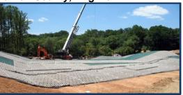
Articulated concrete blocks were placed in the auxiliary spillway.
