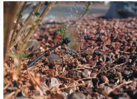
Low pressure sprinkler systems conserve water by delivering small amounts exactly where needed.
