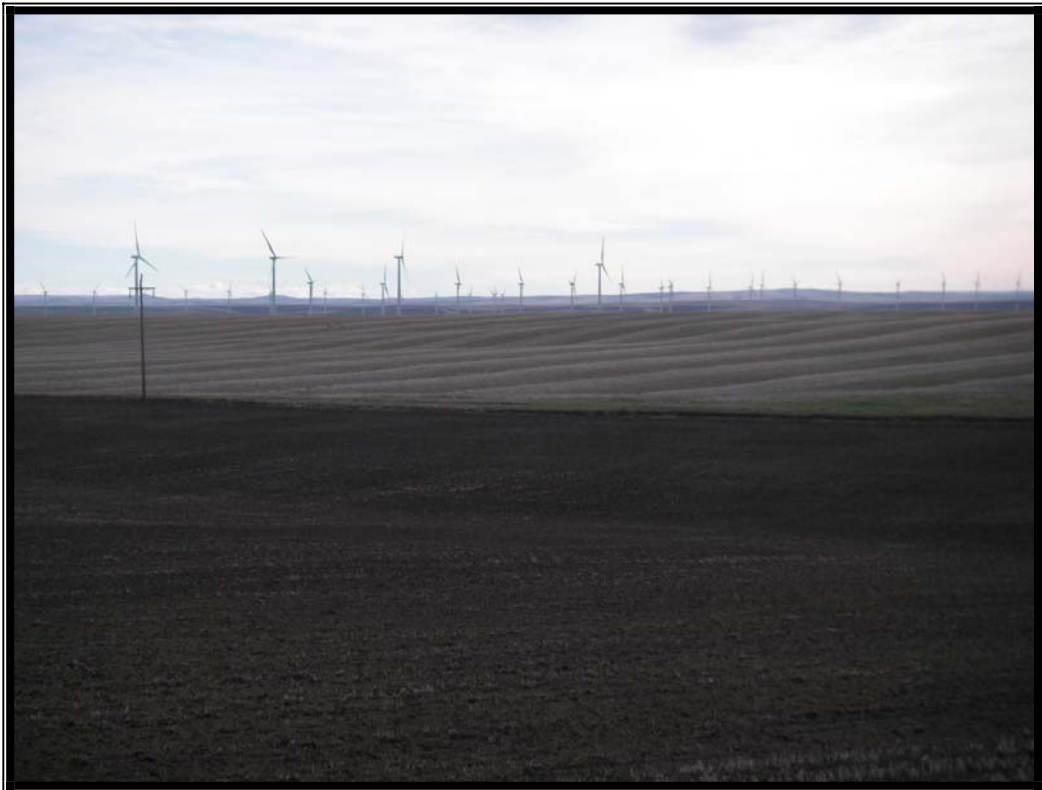
PHOTO 2: Klondike II Wind Project viewed from N. Klondike Road.
