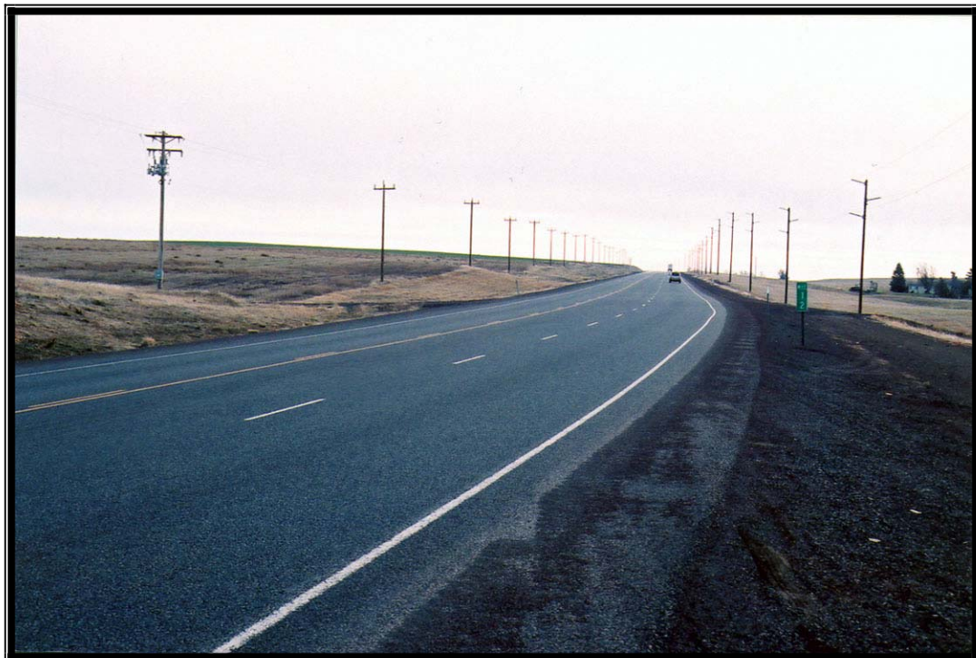
PHOTO 8: US 97 at MP 12 looking south.
