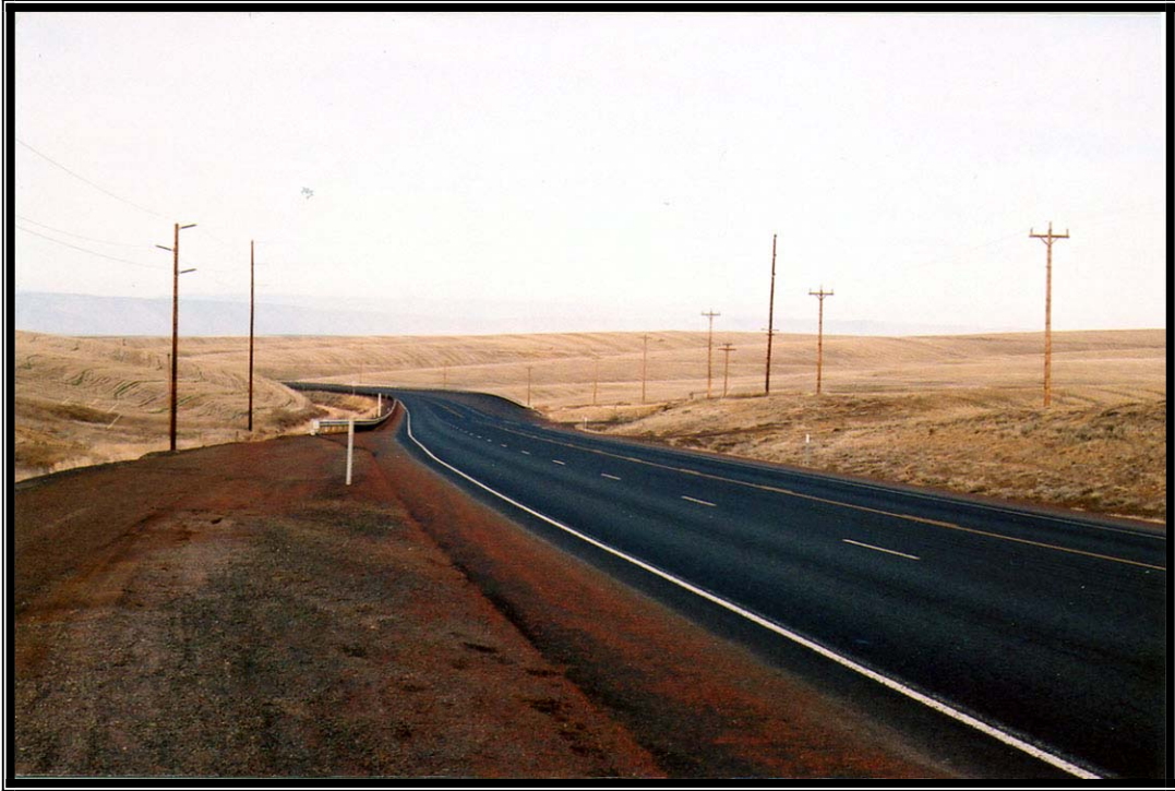
PHOTO 9: US 97 at MP 12 looking north.
