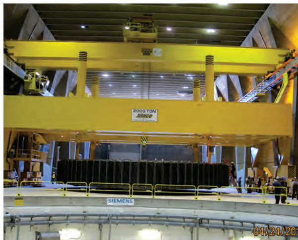
Figure 2: Rotor from the Grand Coulee Dam. Credit: Bureau of Reclamation
