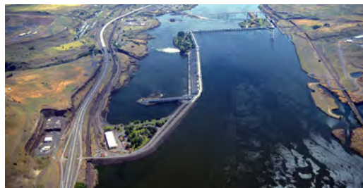
Figure 5: The Dalles Dam on the Columbia River.
