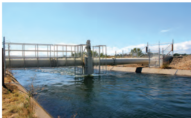
Figure 1: Hydrokinetic Demonstration at Roza Canal. Credit: Instream Energy Systems
