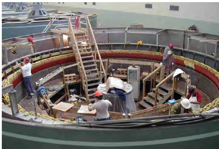
Figure 3: Generator Rewind.
