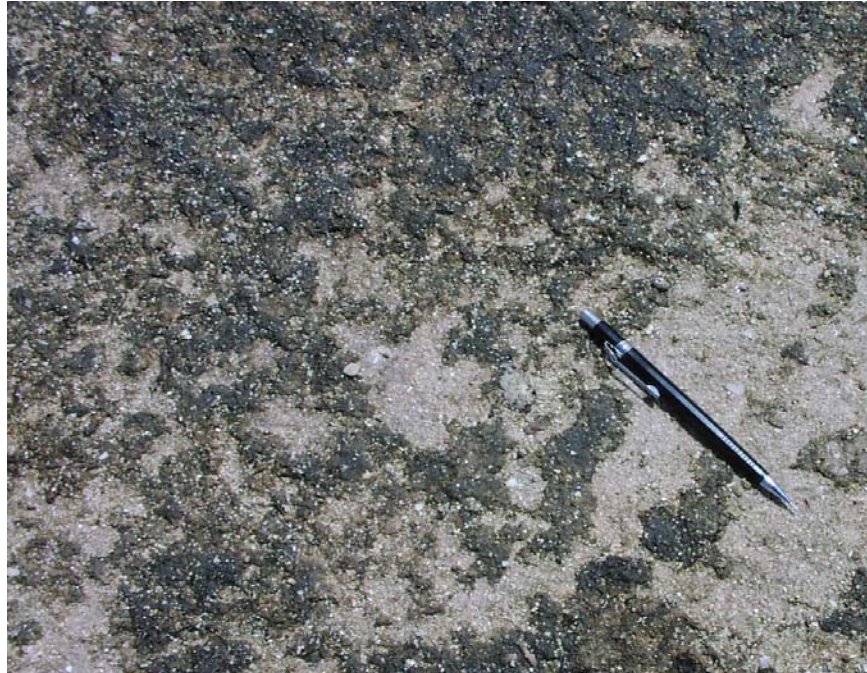
Figure 36. Close-up view of algal crust in a coastal wetland.
