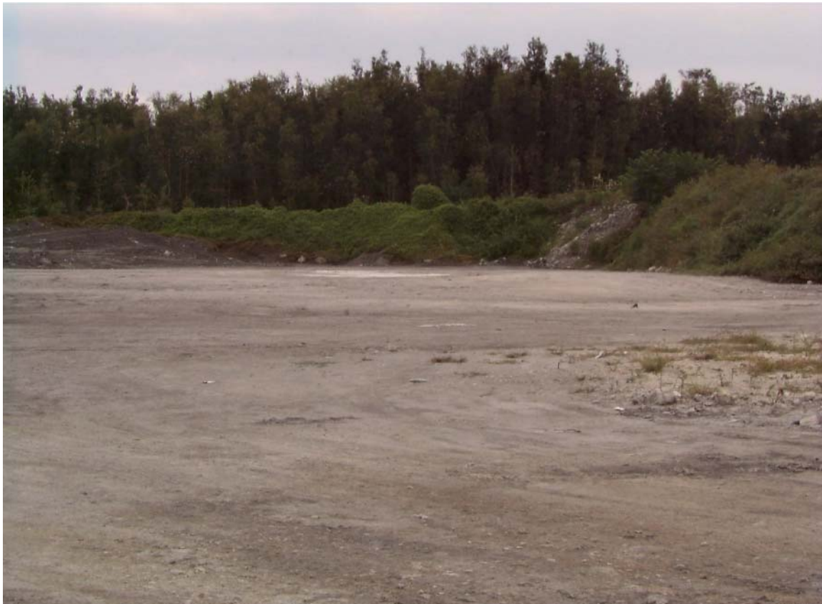
Figure 35. Surface soil texture of rock due to scraping and removal of the natural organic soil
