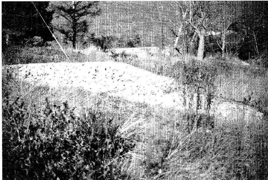
FIGURE 13. GABION SPUR; LOYALSOCK CREEK NEAR LOYALSOCKVILLE, PA.
