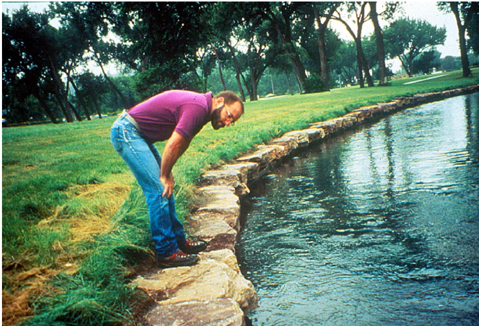
Figure 9. Bank protection and habitat enhancement using stone lunkers, Rapid Creek, Rapid City, SD
