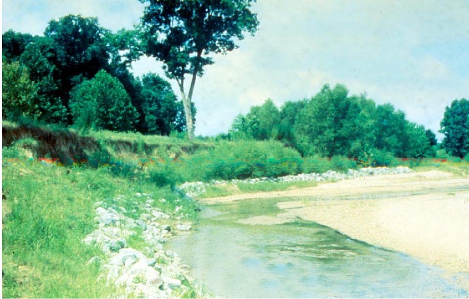
Figure 4. Bank stabilized and revegetated bank, Johnson Creek, MS
