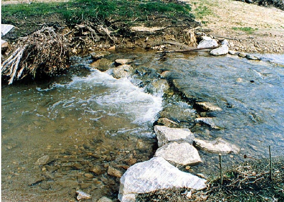
Figure 8. Habitat enhancement with the use of low-flow stone weirs, Paint Branch, MD
