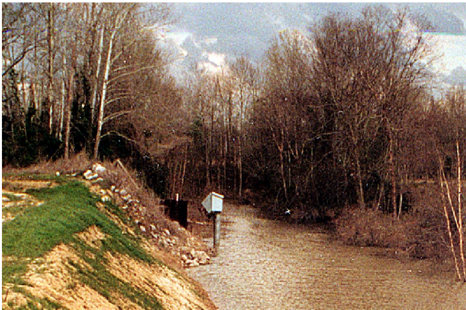
Figure 7. Stable channel upstream from grade control, Hotophia Creek, MS
