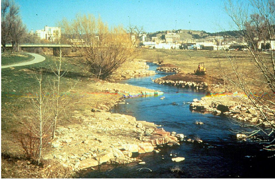
Figure 14. Project designed to provide flood protection, aesthetics, and habitat enhancement, South Platte River, Denver, CO
