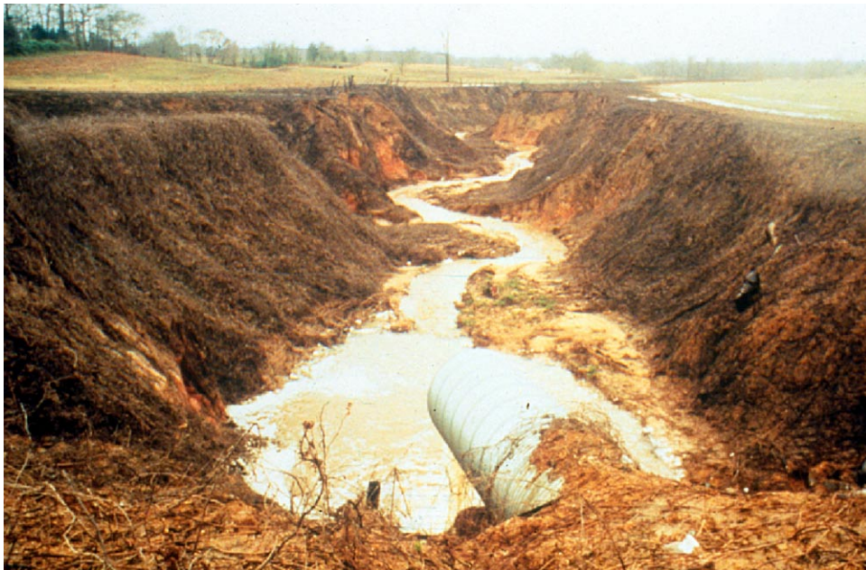
Figure 5. Channel bed and bank erosion due to degradation, Hotophia Creek, MS
