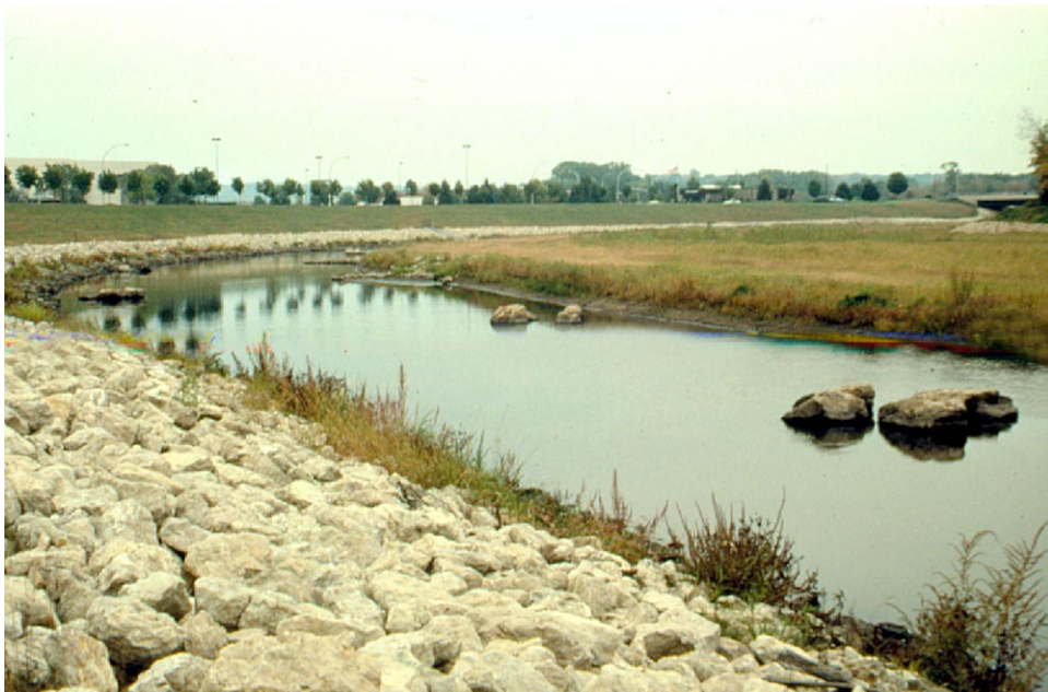
Figure 13. Project designed for flood protection with habitat enhancement features boulder clusters and low-flow deflectors, Zumbro River, Rochester, MN
