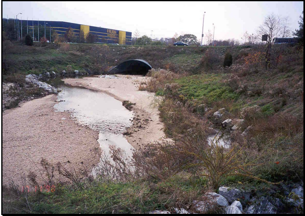
Figure 8.5 Post-project channel changes in Whitemarsh Run, Maryland, November, 1998. Note the channel straightening and sedimentation in the outer-bank meander pool at the head of restored reach.
