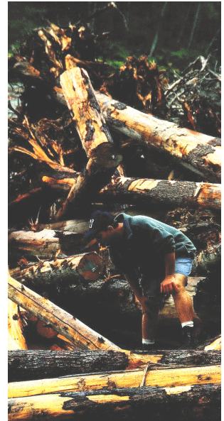
The ELJs are held together with glue (left). Civil engineering graduate student Tracy Drury (right) inspects one of the jams. He analyzes fluid mechanics and calculates the scouring patterns that the team believes will create pools beneficial to fish.
