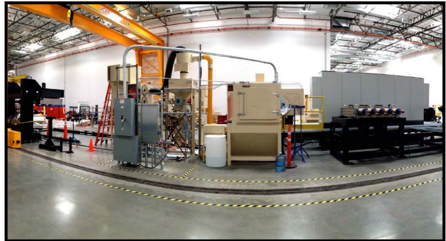
Installation of the first winding station for the central solenoid at General Atomics (San Diego, CA)
