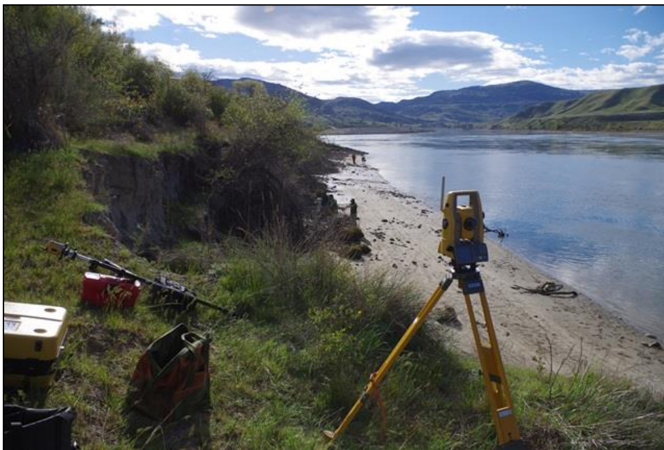
Figure 11. Start of pre-construction data retrieval at 45-OK-196/197, view to east.
