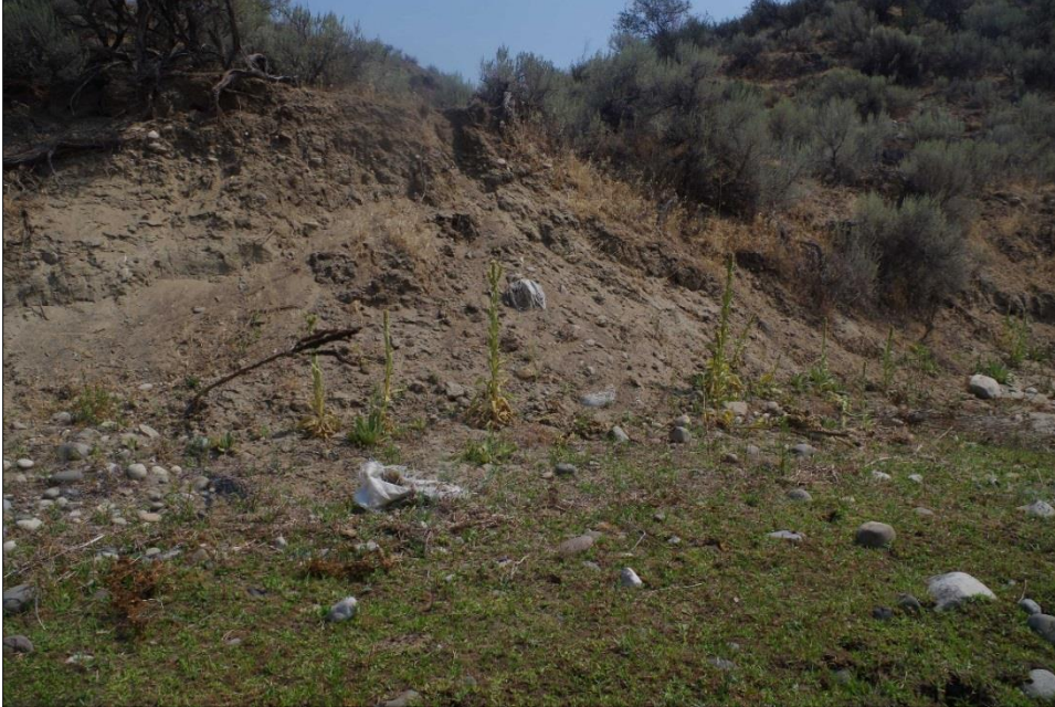
Figure 7. Condition assessment at 45-DO-249 identified cattle trail damage at an early historic privy that was partially excavated about 10 years ago and refilled with the sandbags now dislodged in the foreground. View to east.
