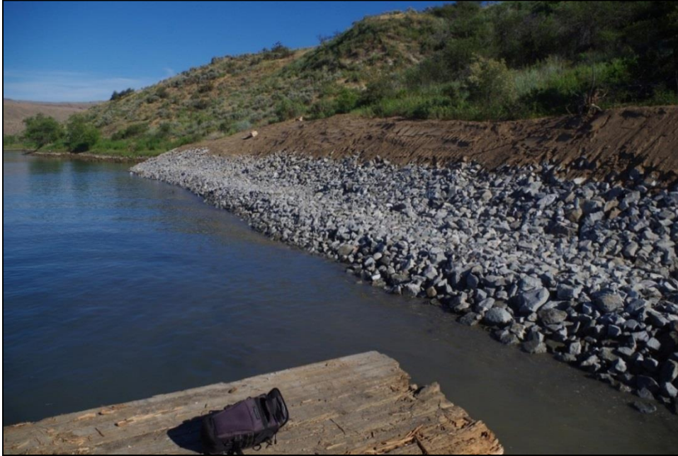
Figure 17. The west-end section completed at 45-OK-196/197; note the shelf mid-slope; fines for planting added to top of slope. View to northwest.
