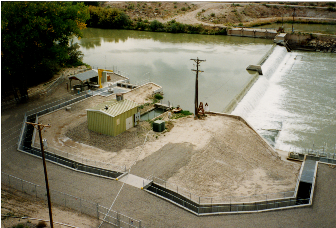
Figure 2—Redlands Conventional Fish Ladder on the Gunnison River, Colorado
