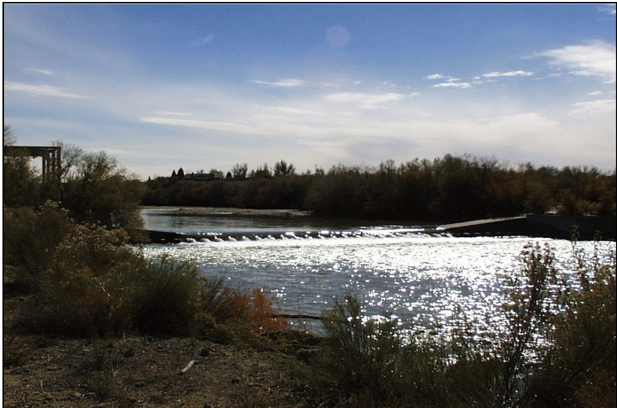
Figure 1 - Public Service Company of New Mexico Diversion Dam
