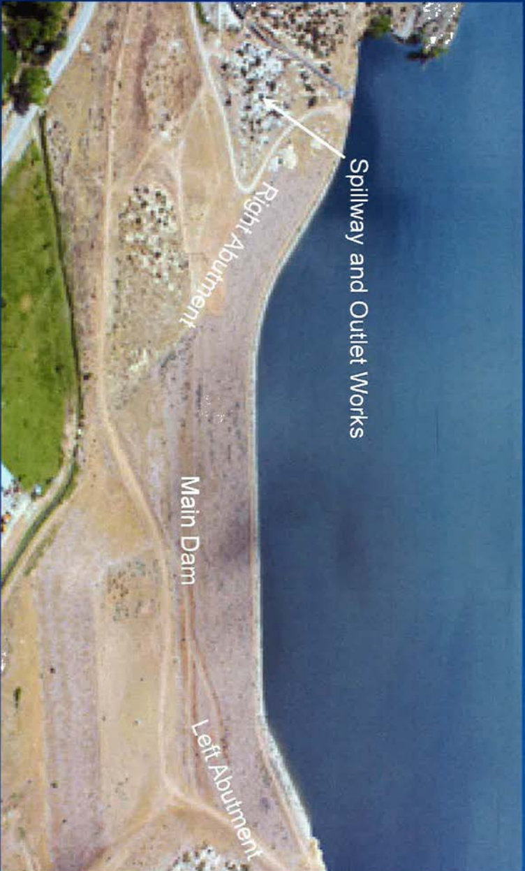
Figure 1. Steinaker Dam is a principal feature of the Vernal Unit of the Central Utah Project. Located approximately 3.5 miles north of Vernal, Utah, Steinaker Dam impounds Steinaker Reservoir, an off-stream reservoir with a total capacity of 40,043 acre-feet at elevation 5520.5 feet., enough to supply two-years' worth of irrigation water.
