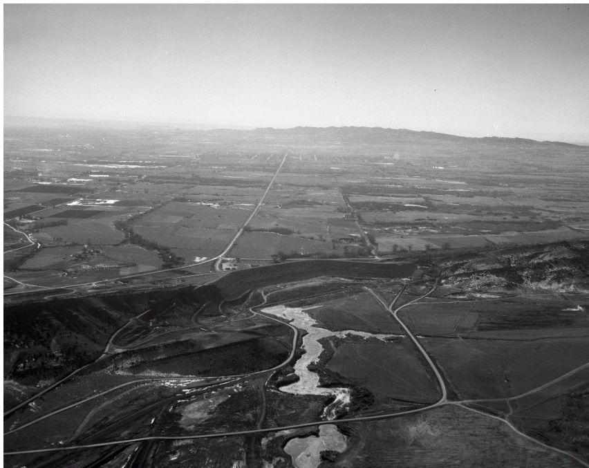
Figure 0.8 Looking south at the completed dam at the upstream face. Project photograph P325-418-0477a, photograph by Stan Rasmussen, 1/18/1961.
