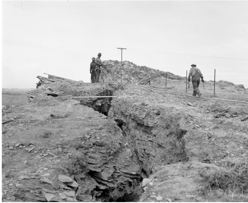
Figure 0.9 View of crack in the left abutment of dam. Workmen are drilling holes for blasting. Project photograph P325-418-1239, photograph by R. H. Felter, April 1966.
