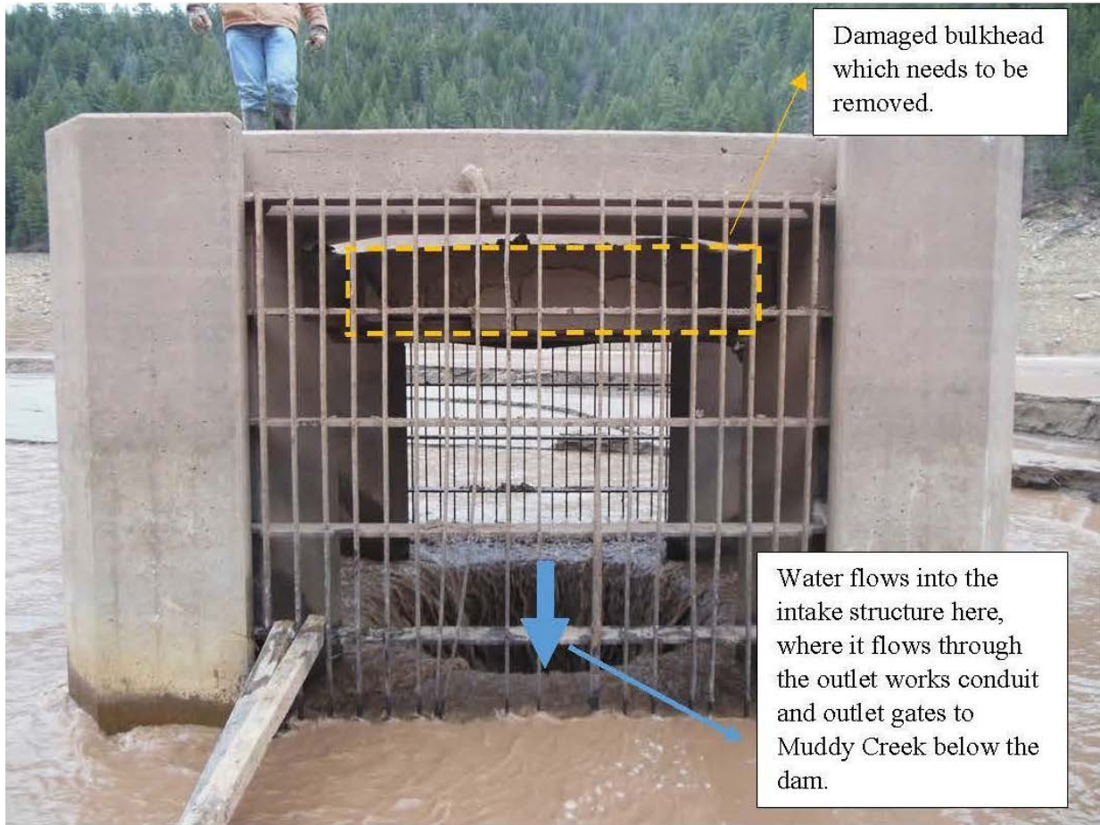
Figure 2. Photo of the intake structure.
