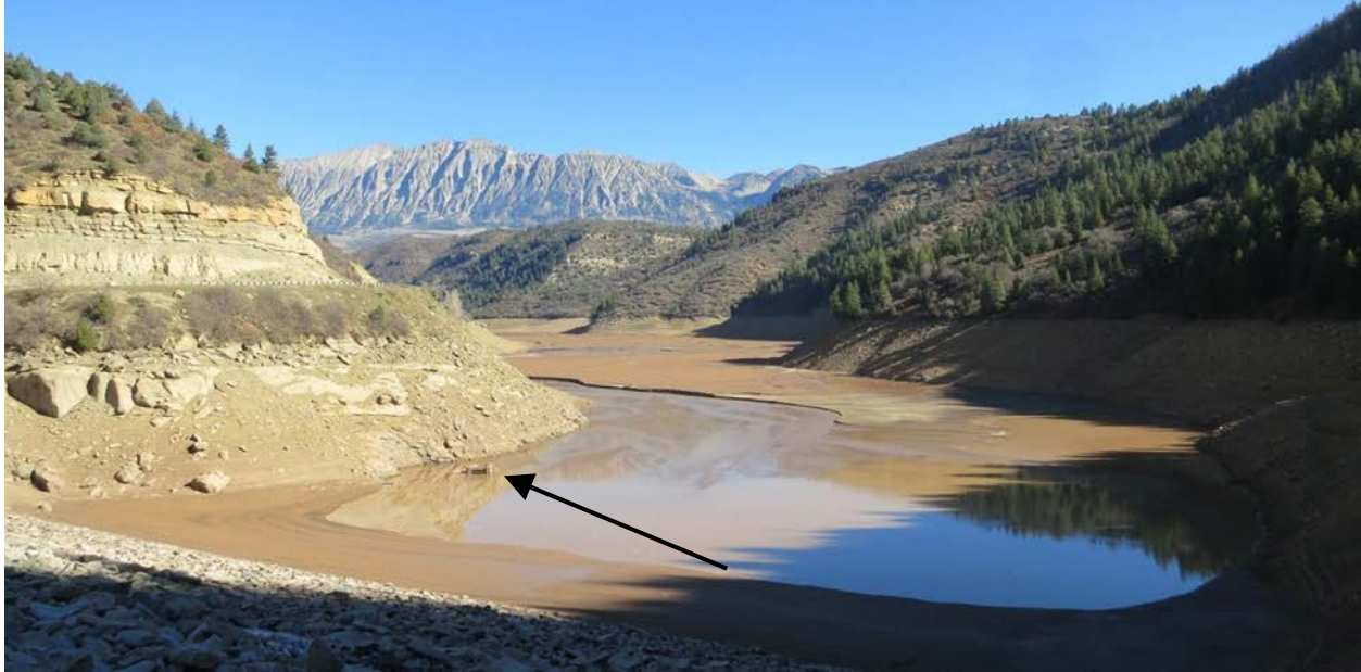
Figure 4. Paonia Reservoir in October 2014, prior to excavation work. The intake structure (black arrow) is nearly buried beneath about six to seven feet of sediment, and sediment has filled the reservoir’s dead pool.
