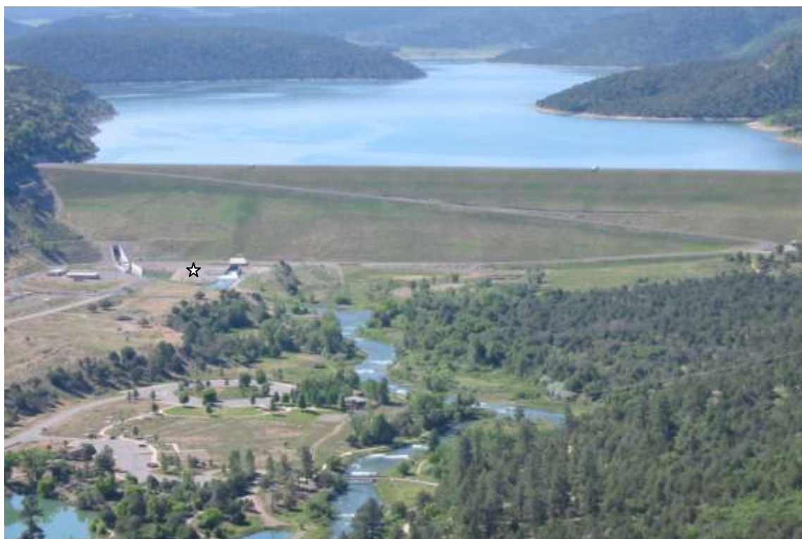
Figure 4. Looking south across the day use area toward Ridgway Dam. Star shows approximate powerplant location.
