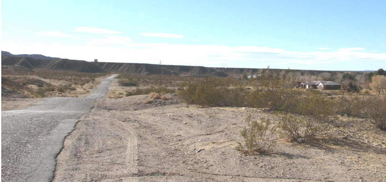
Photo 7 (KOP 39). Viewing south on New Gold Butte Road where the 7-year transmission line would cross the road (216°).
