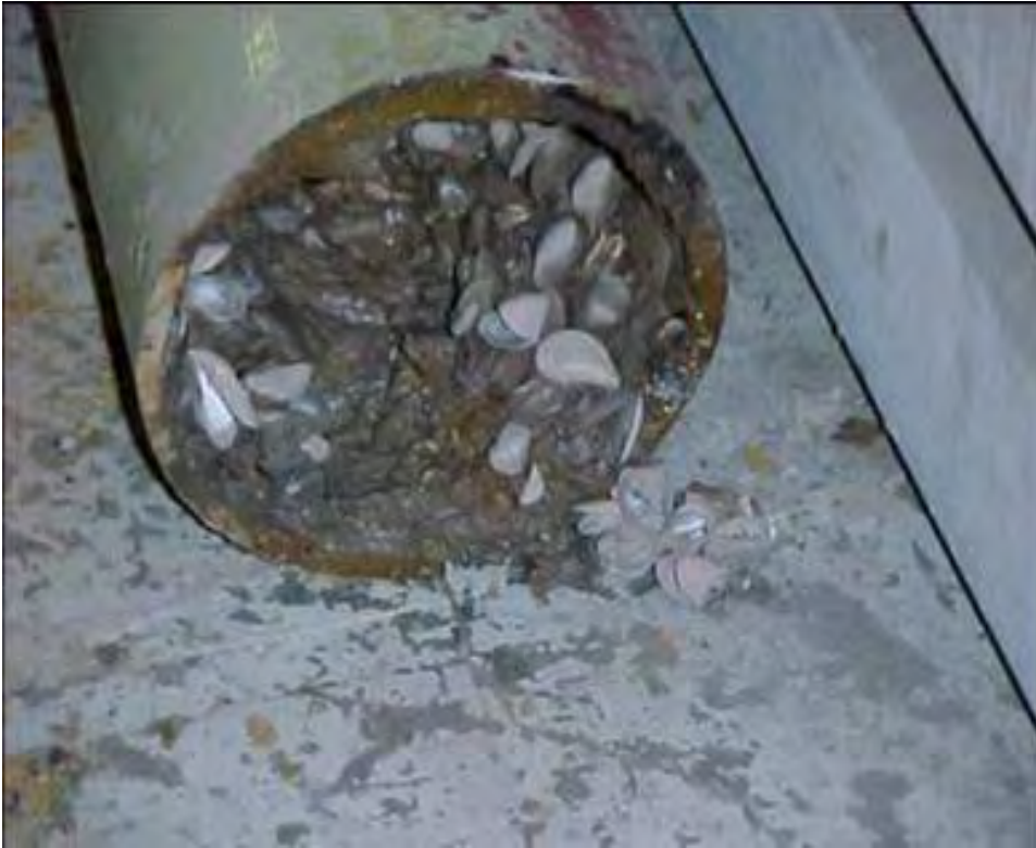
Figure 3. Clogged pipe.
