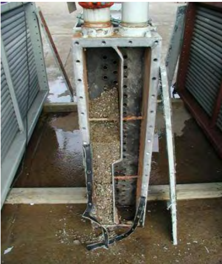
Figure 2. Dead mussel debris in cooling unit.
