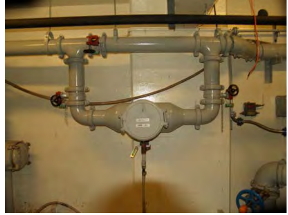
Figure 7: Bypass System
