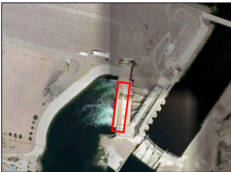
Figure 5. Aerial photo of Davis Dam showing the 5 generators inside the red box.
