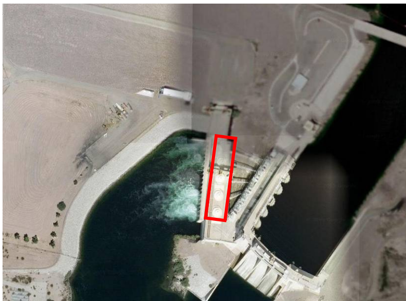
Figure 4. Aerial photo of Davis Dam showing the 5 generators inside the red box.
