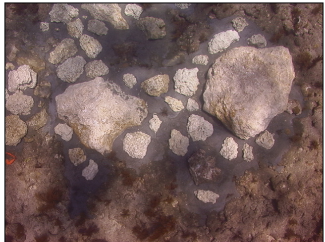
Figure 9. Completed restoration with reef restoration modules (left) and "puddle pour" with boulders (right) each surrounded by limestone "dressing" stones (photo credit: Coastal Planning and Engineering, Inc.).
