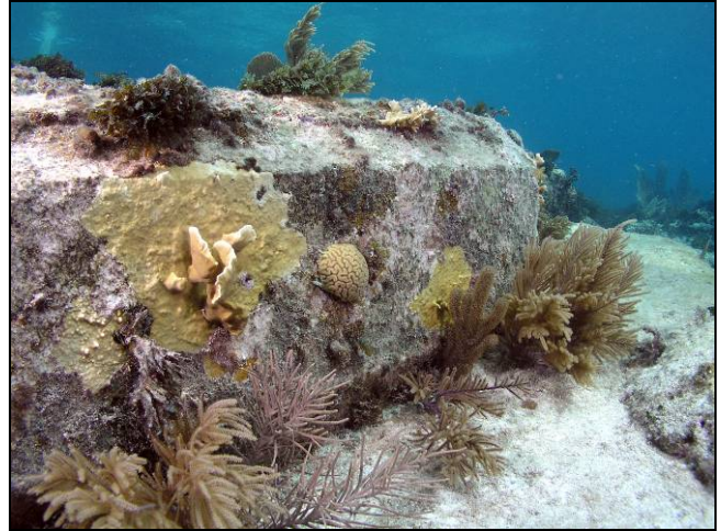
Figure 14. Restoration armor units showing biological condition 10 years after installation (photo credits: Jeff Anderson NMSP/NOAA).
