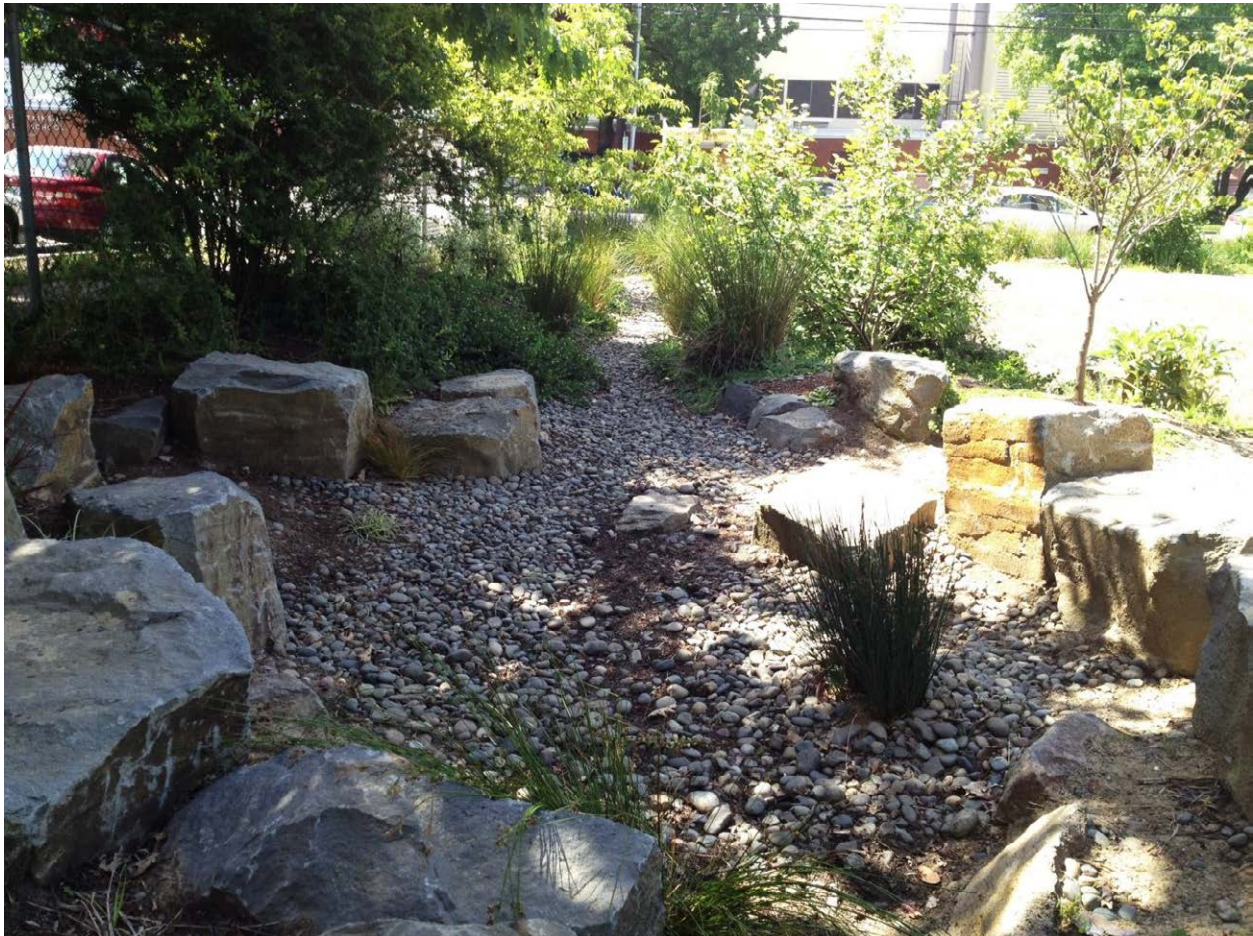
Bioretention area with low-maintenance plantings and hardscape (Photo credit: M. Frey)
