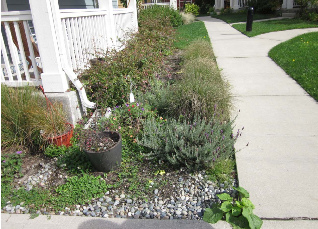
Residential downspout disconnection in Seattle, WA
