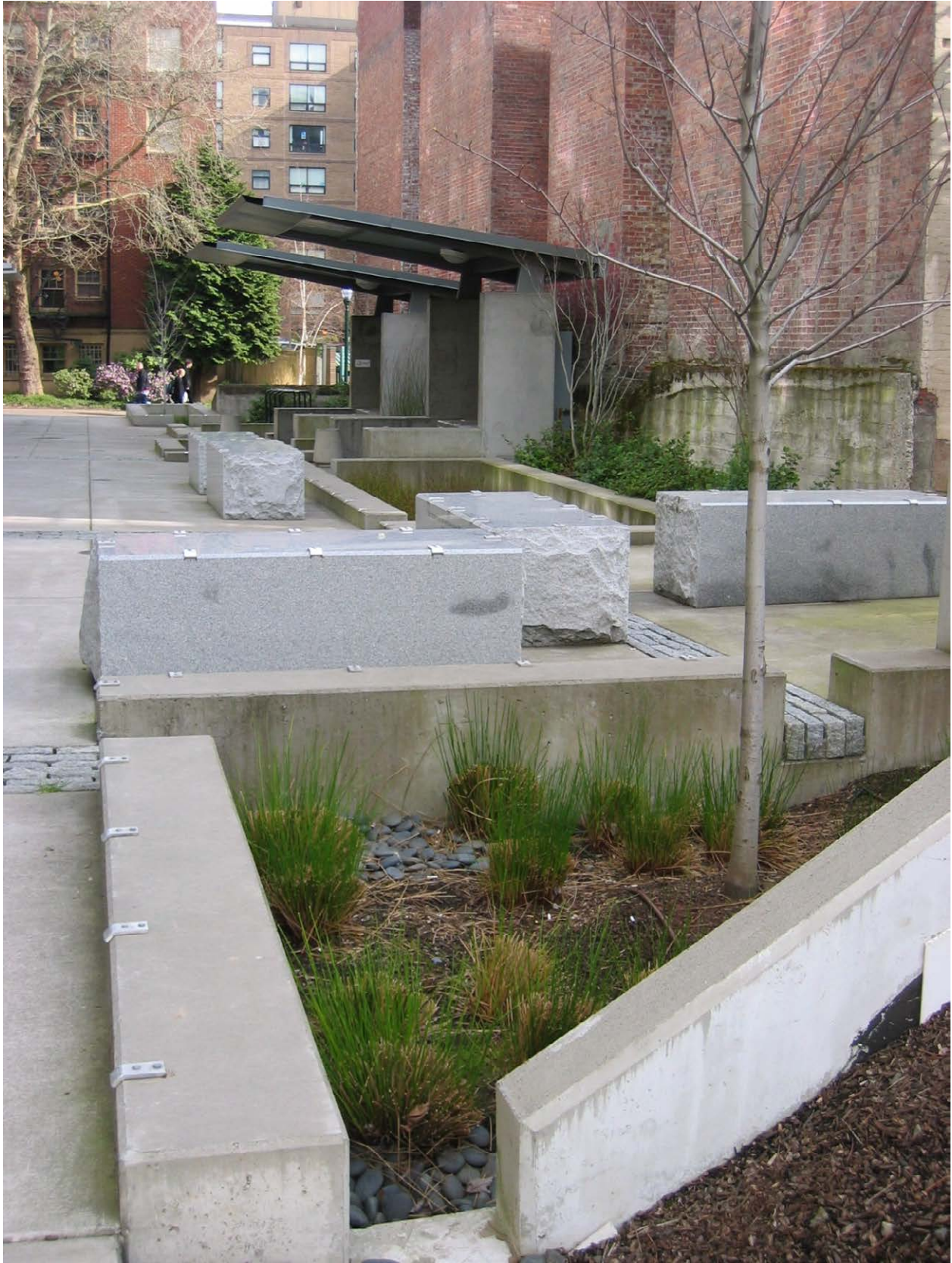
Bioretention in a plaza gathering space in Portland, OR (Photo credit: M. Frey)
