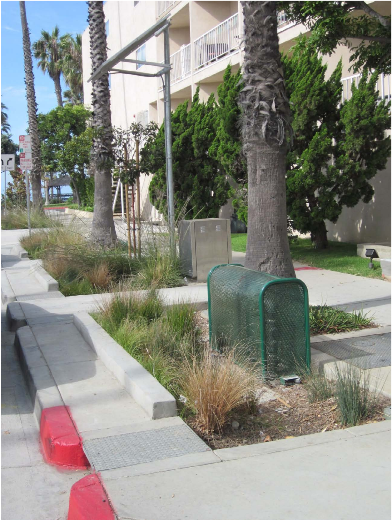
Bioretention sidewalk retrofits in Santa Monica, CA
