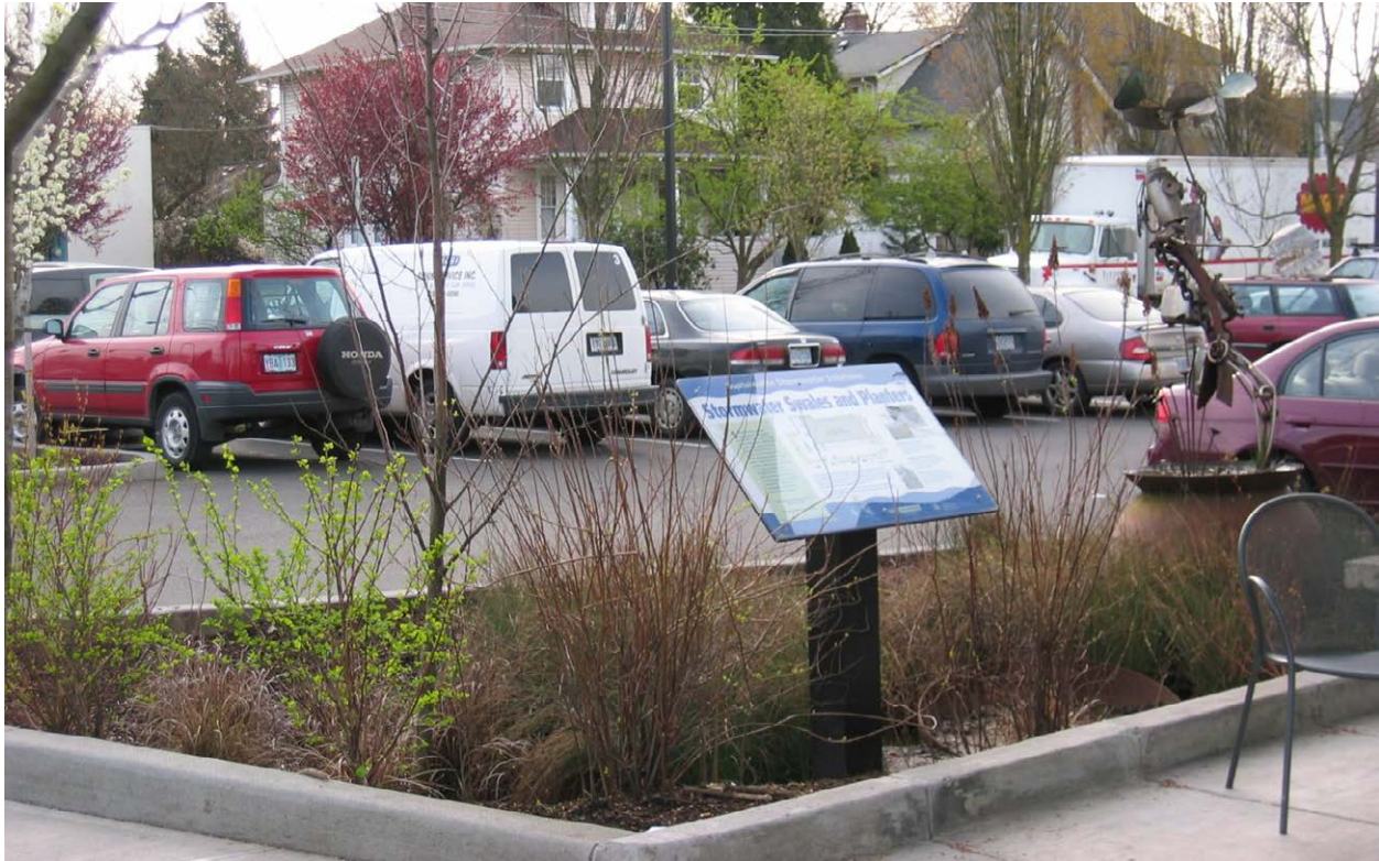
Signage describes the purpose and functions of a bioretention area, Portland, OR (Photo credit: M. Frey)
