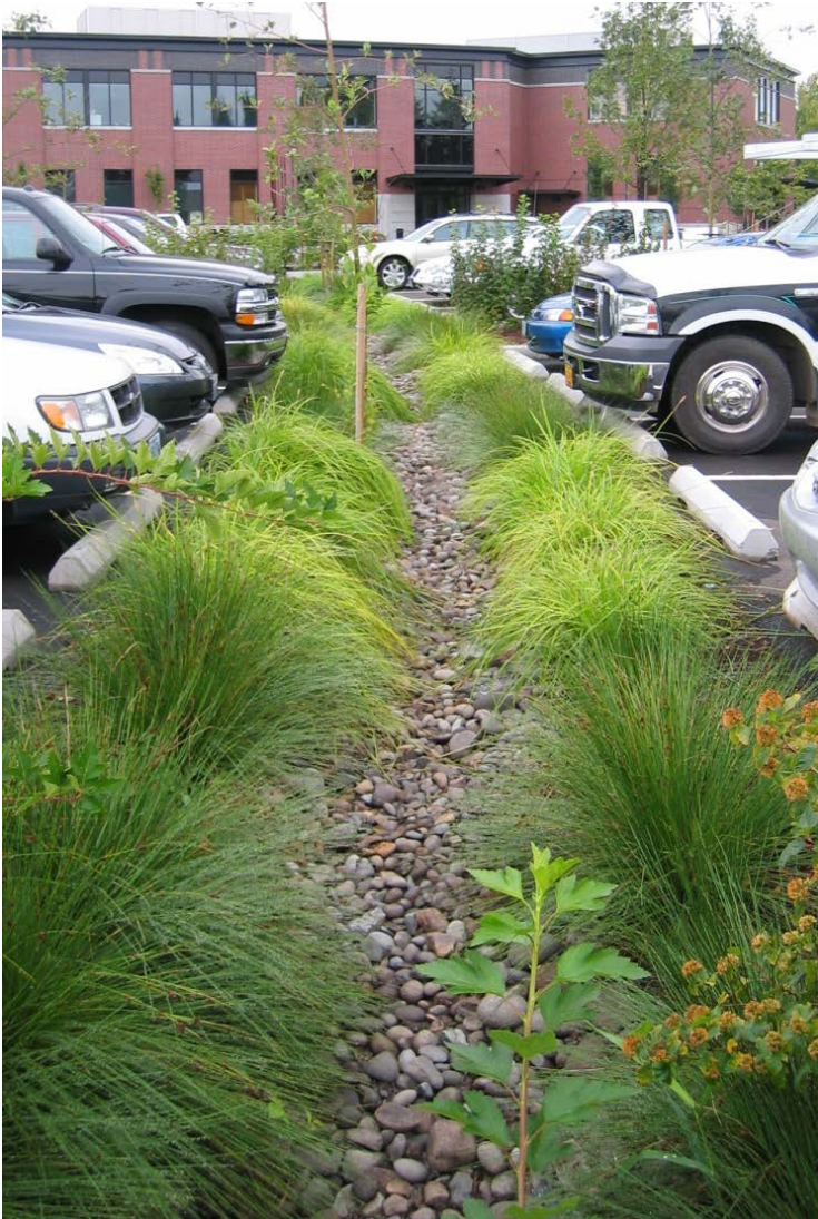
Parking lot bioretention, Wilsonville, OR (Photo credit: M. Frey)
