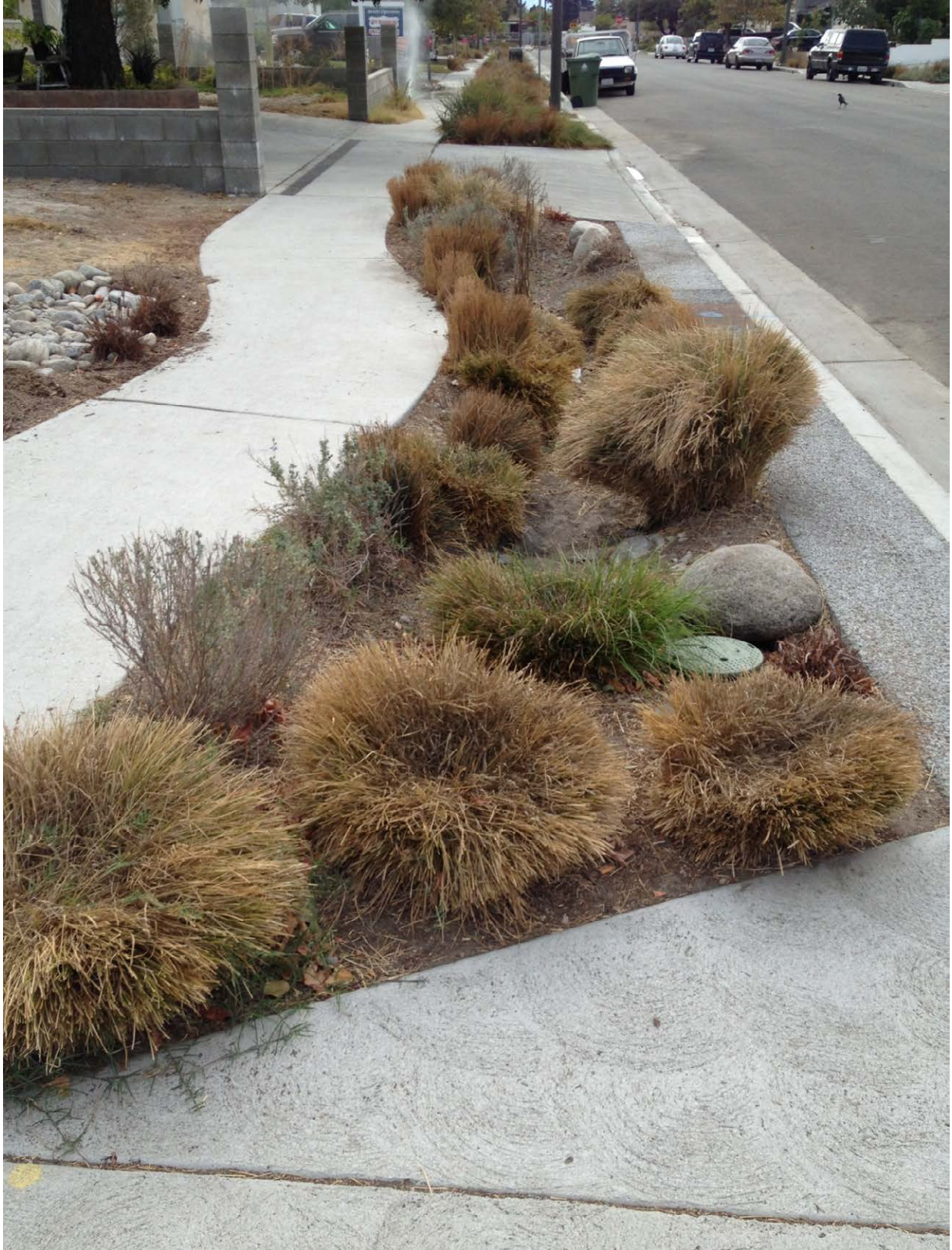
Bioretention with xeriscape incorporated into the right-of-way, Los Angeles, CA (Photo credit: Tetra Tech)
