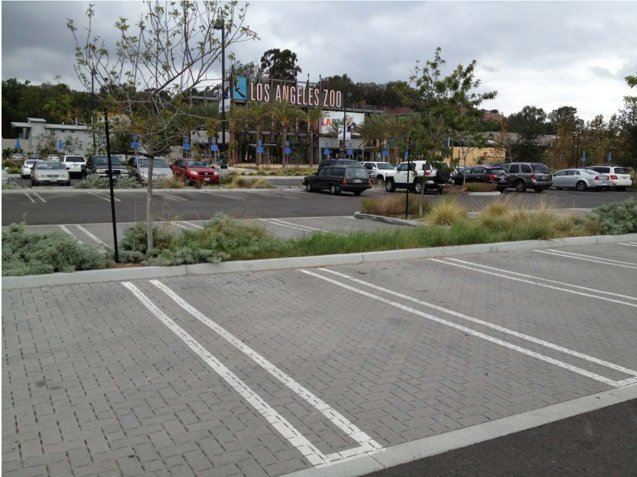
Porous pavement parking stalls and bioretention at the Los Angeles Zoo (Photo credit: Tetra Tech)
