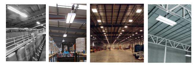
These measures are for HO Linear Fluorescent Hi-Bay lighting systems. This measure series is designated by replacing baseline of >250 watts with linear fluorescents with HO ballasts. All HO T8 lamps and ballasts must meet CEE high performance requirements to be elligible. Also, lamp mounting heights must be greater than 15 feet. The 6 lamp T5 is considered a non-standard measure. Utilities and Trade Allies are encouraged to use controls with this application.
