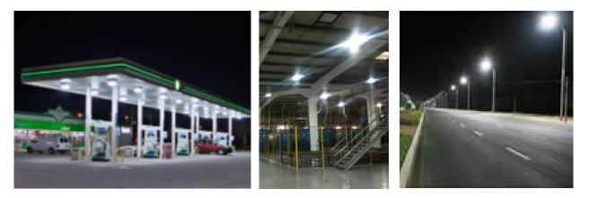
These measures cover induction lighting including screw-in and hardwire fixtures. All induction products must have a lamp life of >60,000 and a CRI >60. Induction retrofit kits can be used but are not recommended by BPA.
