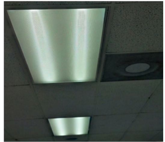
These 2'x4' troffers with acrylic lenses (above) originally had 3 fluorescent T12 lamps, and now have 2 T8 LED linear replacement lamps that create white and gray stripes on each troffer lens. With a new lens designed for LED's, each troffer would have a more uniform appearance.
