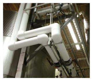
400 Watt High Pressure Sodium (HPS) lighting was retrofited to high performance T-5, and glycol piping insulation was intalled. Ste. Michelle Wine Estates can expect to see a simple payback on their energy bill, after utility rebate, of less than three years for both projects.
