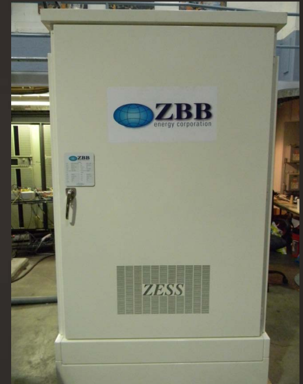
Zinc bromide flow cell battery
