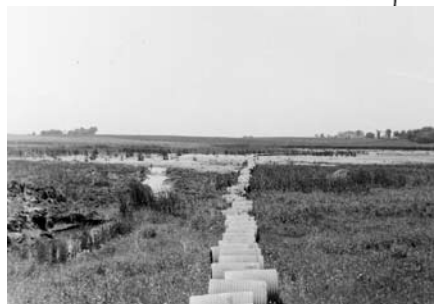
Installation of subsurface tile for wetland drainage in Iowa, circa 1950. Photo courtesy of USFWS.
