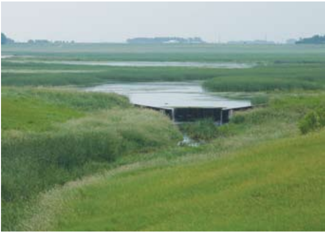
Figure 66. A wetland restoration (re-establishment). This former wetland basin had been completely drained and reclassified as upland. Photo courtesy of South Dakota State University.
