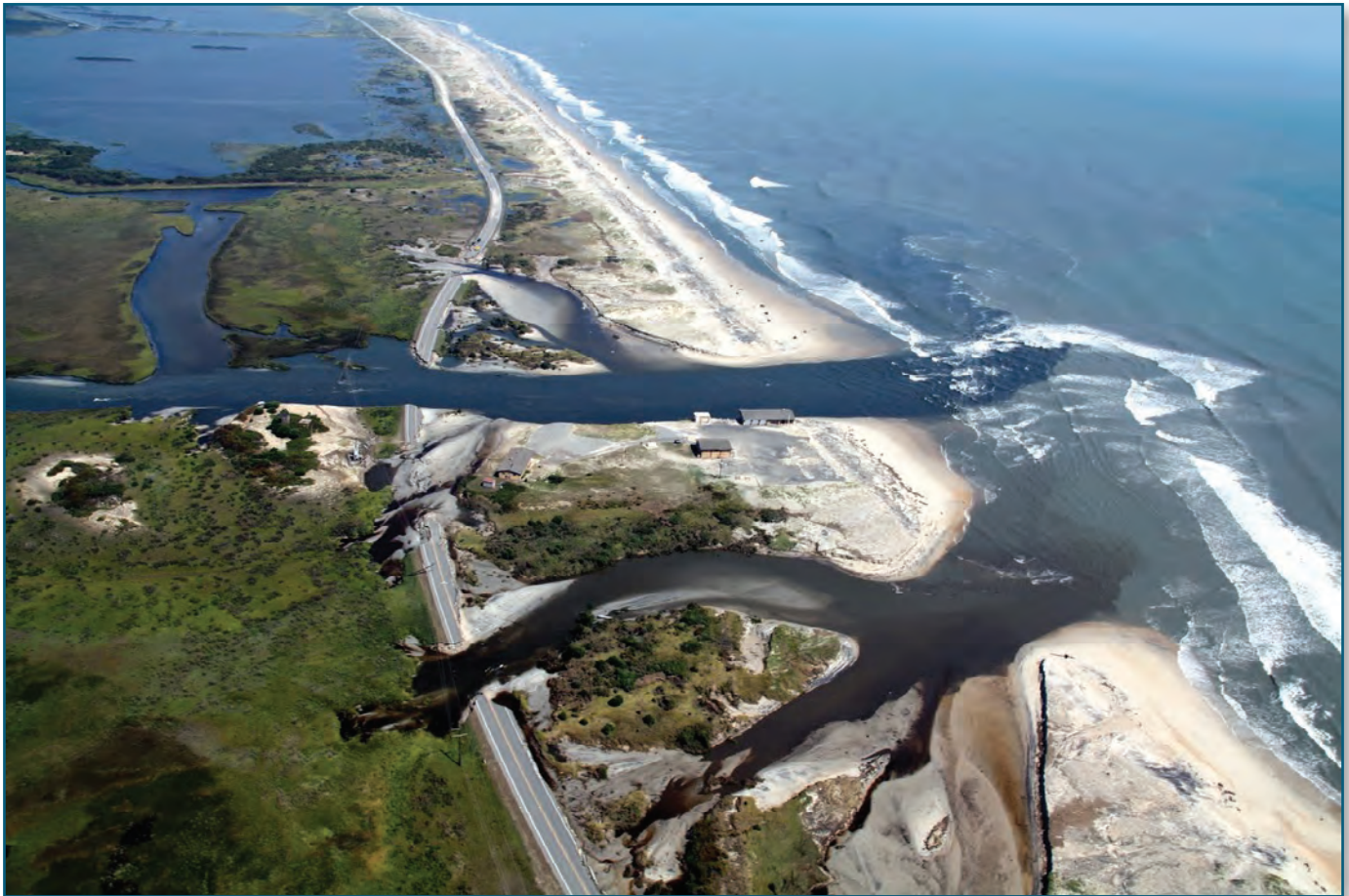
Figure 5. Storm damage and saltwater inundation resulting from Hurricane Irene along the coast of North Carolina, 2011. 8 In addition to the property damage and threats to coastal residents, the frequency and intensity of coastal storms can also influence coastal wetland types and distribution through erosion, deposition of sediments or by increasing salinity.
