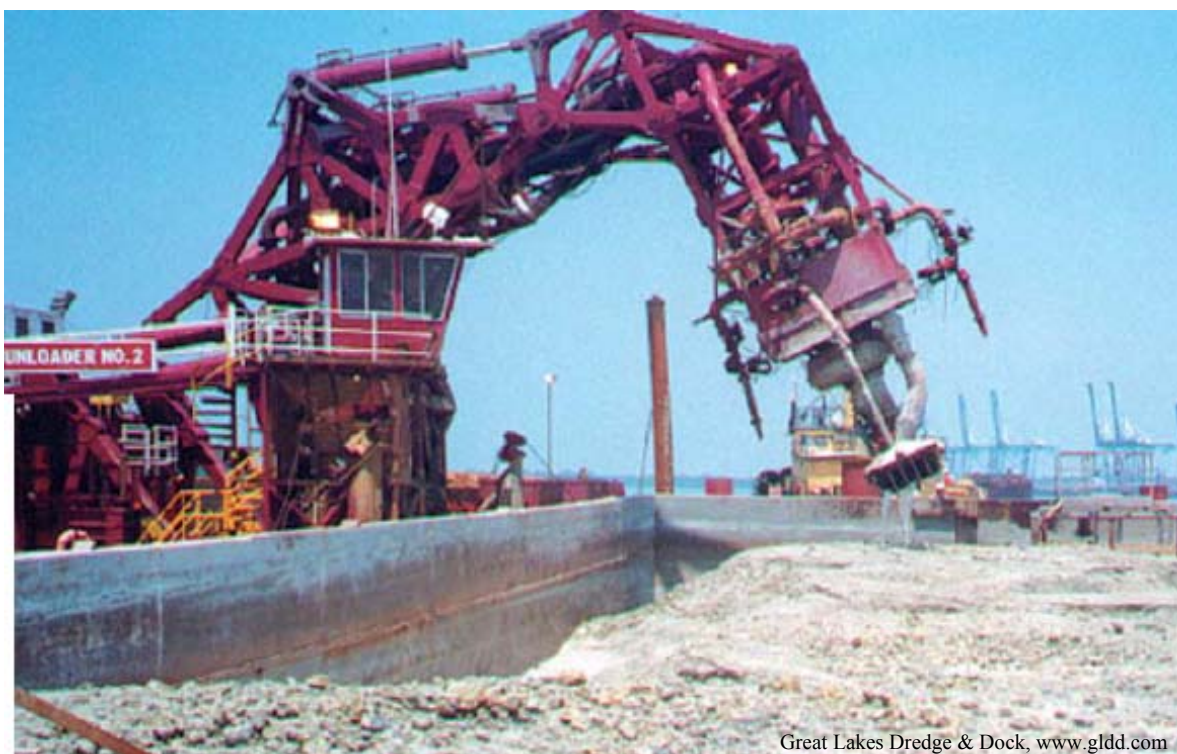
Figure 11. Dredge Material Scow Being Unloaded at a Fill Site
