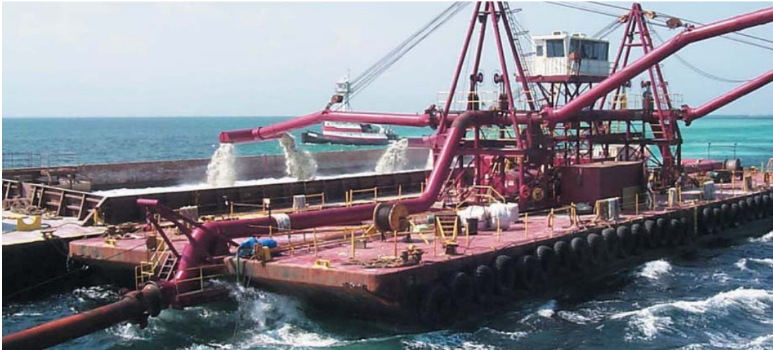
Figure 6. Close-up of Barge Loading Process (the vessels at the top of Figure 5)
