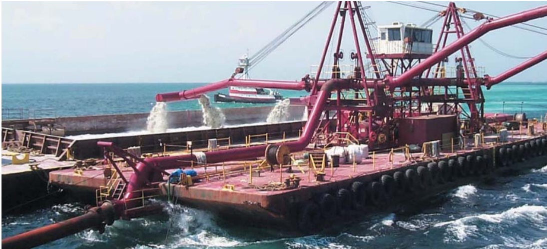
Figure 6. Close-up of Barge Loading Process (the vessels at the top of Figure 5)
