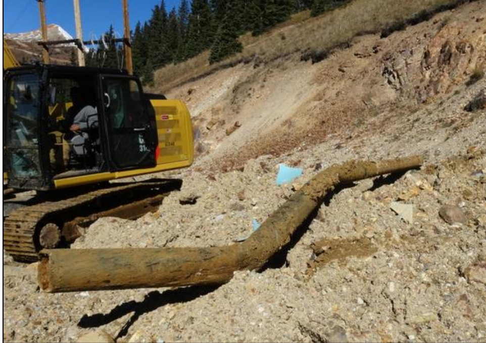
Part of the stinger, following removal in 2014. Source: Environmental Restoration.
