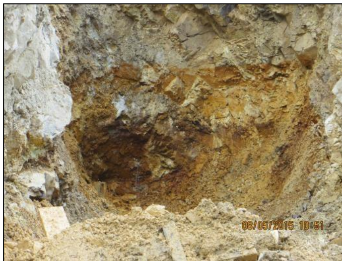
The initial spurt of water from the adit appears in the excavated area, just below a white mark on the rock face. The plug is no longer visible because EPA backfilled the excavation. Source: EPA.
