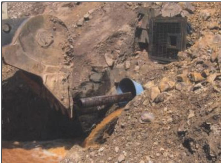
DRMS drives the stinger through the drainage pipe in 2009. Source: DRMS.
