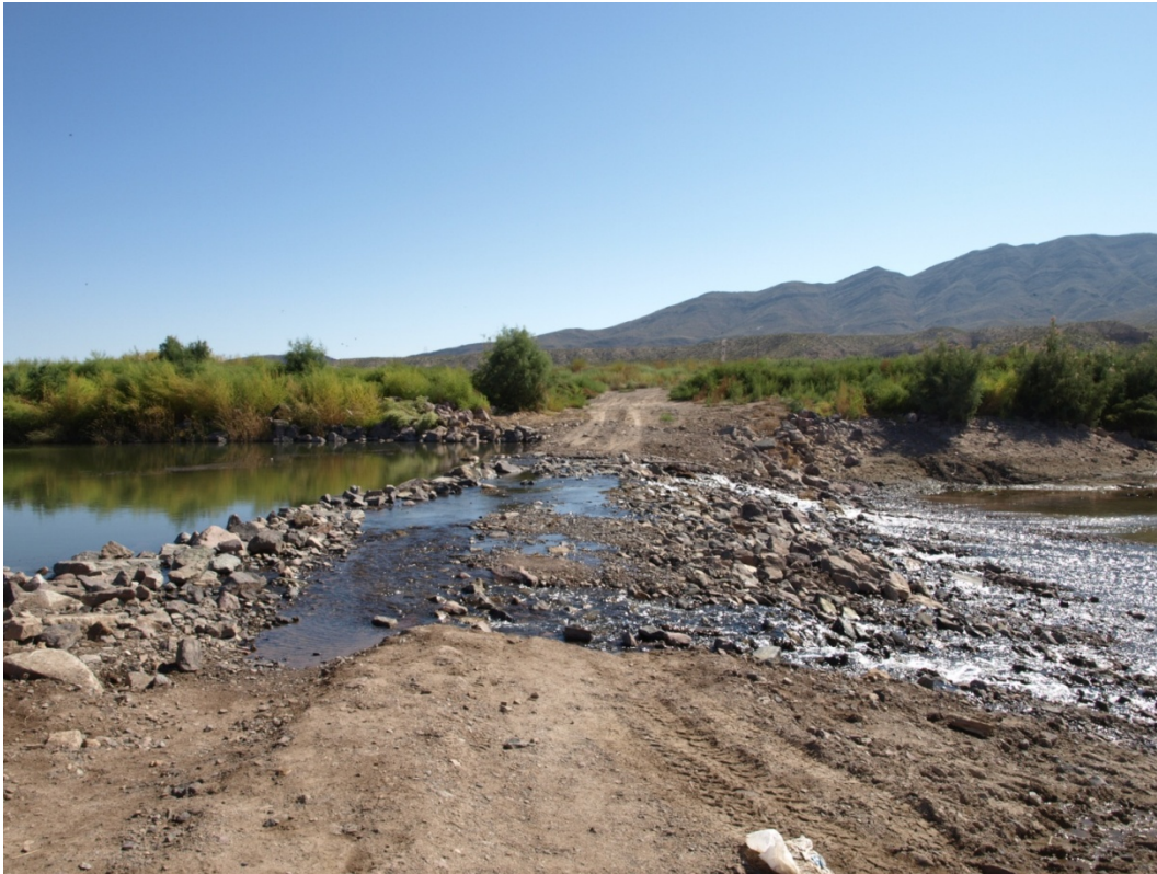
Photo 10: Temporary dike installation on the Rio Grande (October 2012, AuBuchon)
