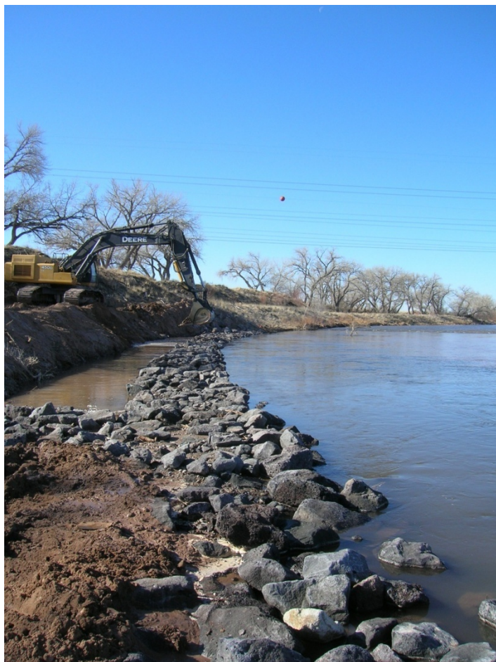
Photo 7: 2012 construction on the LFSTP with tiebacks (March 2012, Mims)
