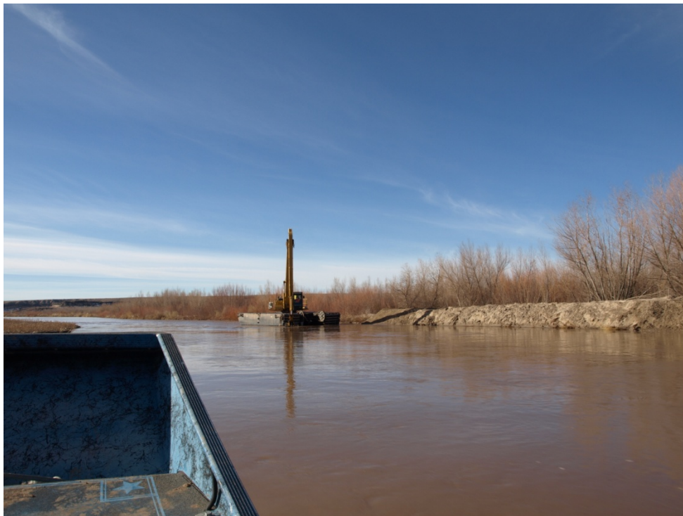
Photo 1: Amphibious excavator working on west berm of the Temporary Channel (January 2012, Casuga)
