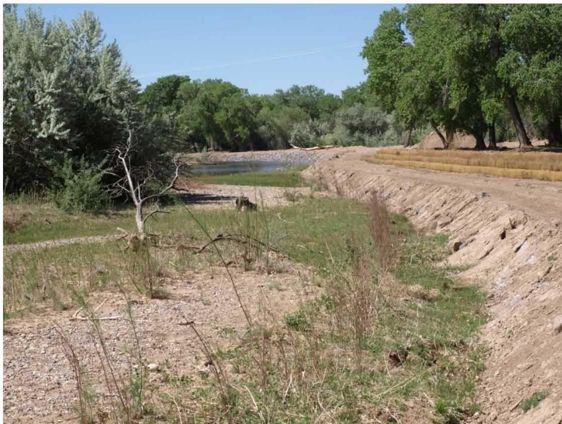
Photo 6: Coyote willow whips, rock toe, and Bio-D blocks at Priority Site RM 212.0 (May 2012, Walton)
