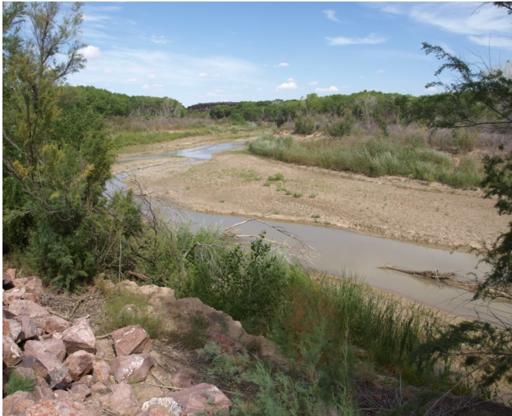
Photo 9: Fort Craig Bend, looking upstream with riprap window in left corner (September 2012, Holste)
