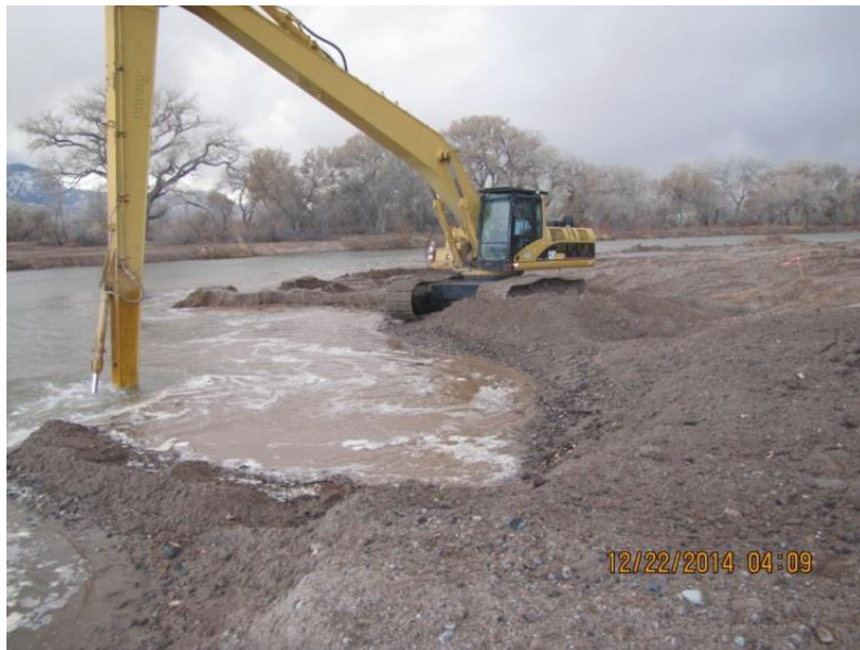
Figure 11: Bar excavation on west floodplain (December 2014, Bui)
