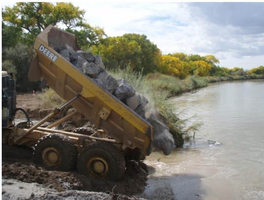
Figure 10: Placement of riprap for bendway weir (October 2014, Bui)
