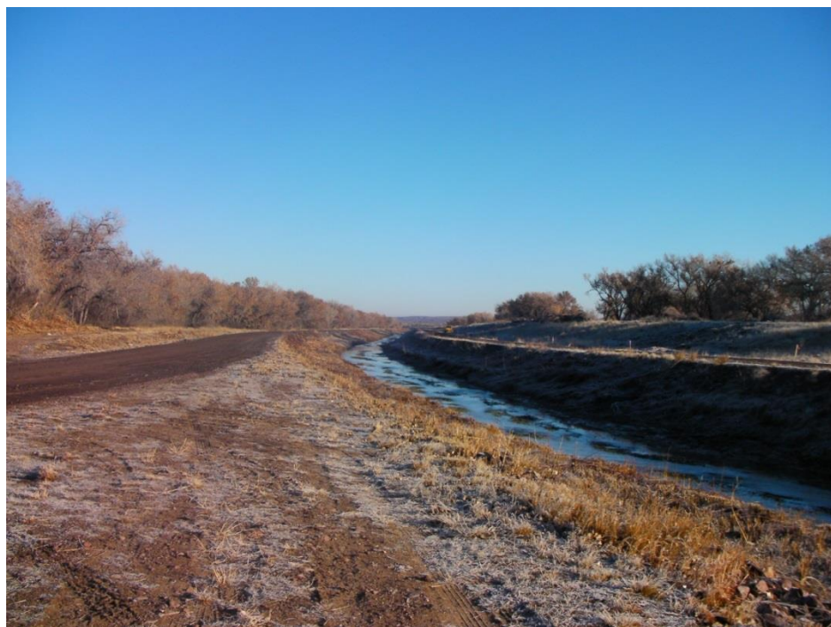
Figure 5: LFCC mowed areas at Otero Bridge (Jan 2015)
