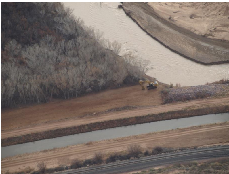
Figure 12: Construction on Phase 3 at the Drain Unit 7 Priority Site (December 2014, AuBuchon)
