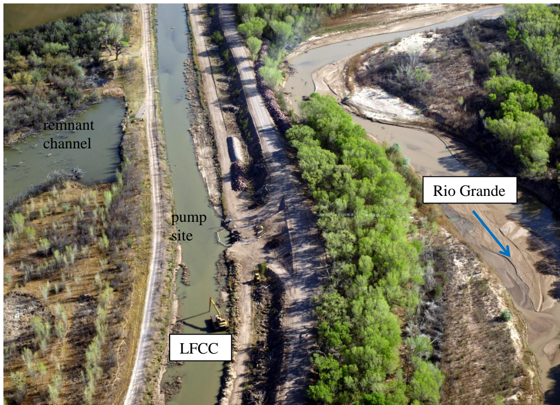
Photo 10: Fort Craig Bend, looking north at the Bend, pump site, and LFCC (April 2013, Holste)
