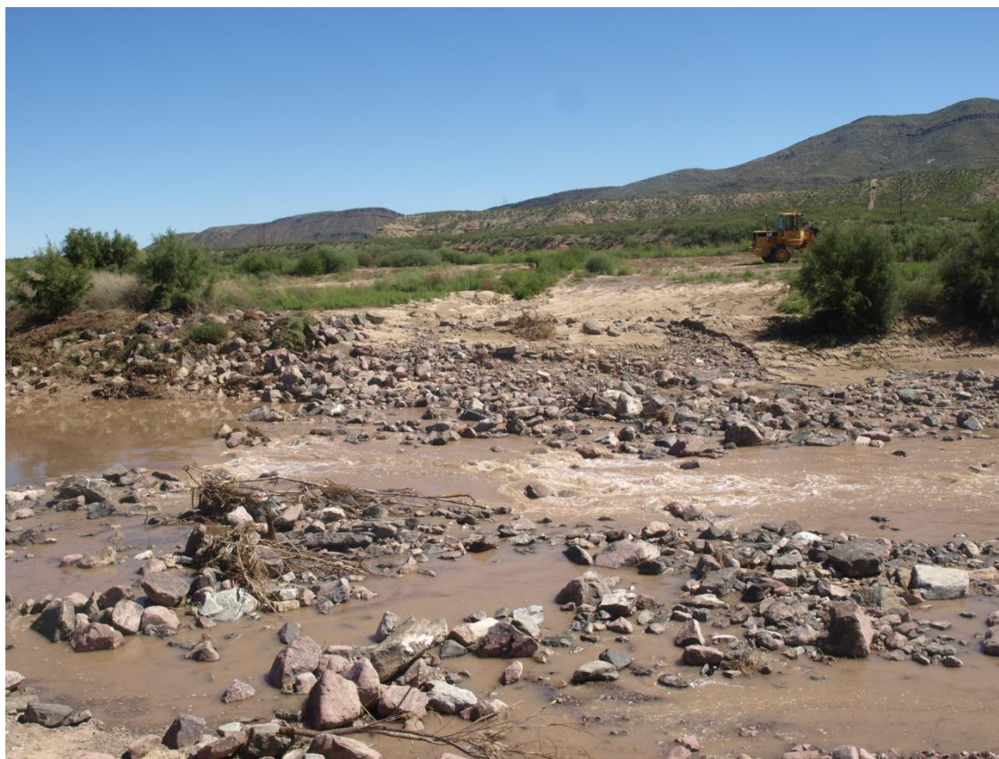
Photo 11: Temporary dike taken out by monsoons in 2013 (September 2013, AuBuchon)
