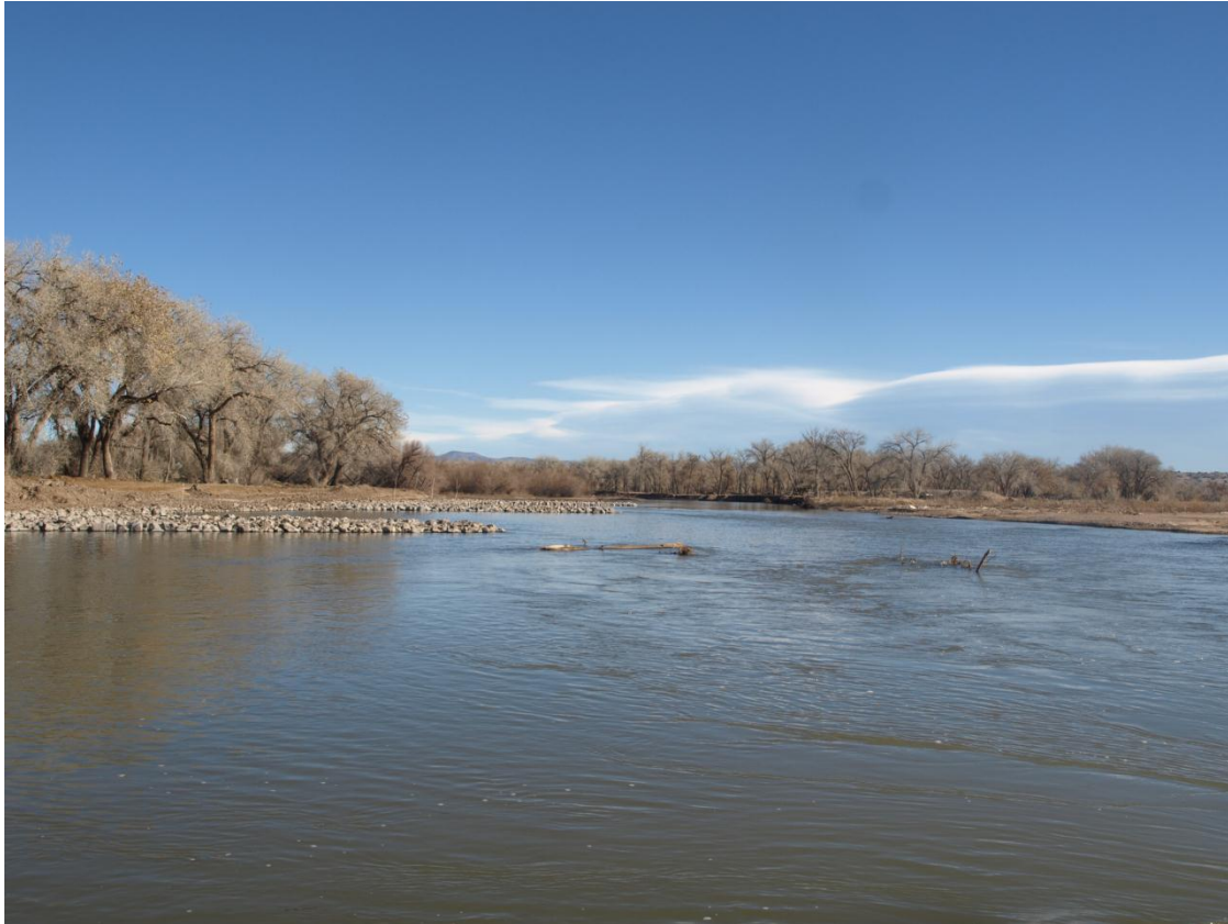
Photo 5: Constructed bendway weirs and longitudinal stone toe with bioengineering at Santo Domingo RM 224.6 (January 2014, S. Benoit)
