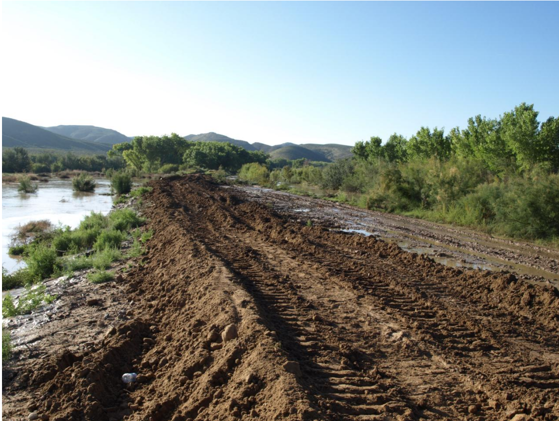
Photo 8: Temporary fix of spoil levee between Drain Unit 7 Extension and the Rio Grande (September 2013, AuBuchon)
