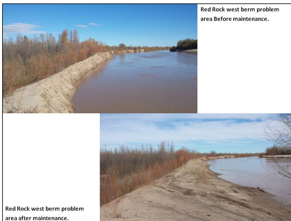
Photo 1: West side berm below Red Rock, before and after maintenance
