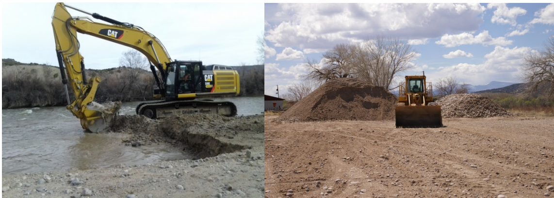
Photos 4 & 5: Sediment deposits excavated and stockpiled (Bui 2015, Gonzales 2015)
