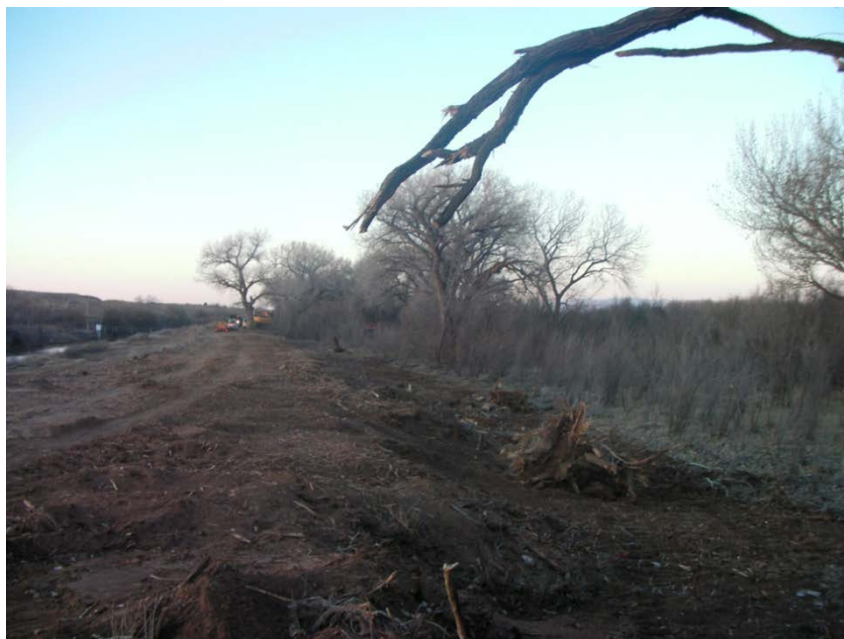
Photo 2: Lower San Juan Riverside Drain Vegetation Removal (April 2015)
