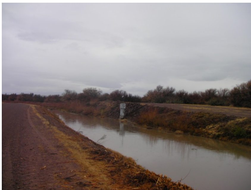
Photo 3: LFCC Vegetation removal at San Marcial Gaging Station (April 2015)
