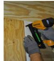
Prime and replace interior trim and, if needed, sill
