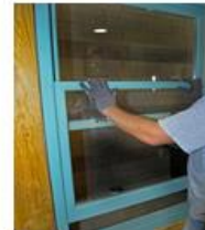
With window secured in place, check for proper function
