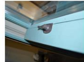
Check that sash locks align properly, indicating window is plumb
