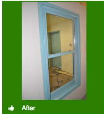
Double pane unit installed with trim in place
