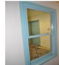
Replace exterior trim and patch exterior siding or finish as needed
