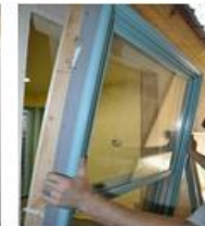
Flanges have been folded out to allow for easy installation
