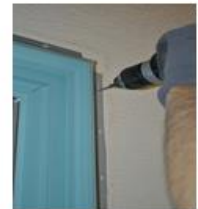
Fasten window flange securely around exterior of entire window
