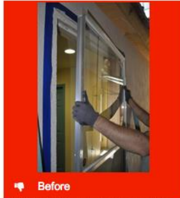
Single pane window is being removed to install double pane unit
