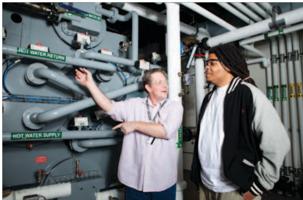
Getting first-hand experience with an adsorber heating and cooling system.
