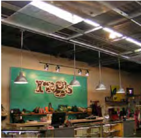
The 4-Lamp LED lighting that Rags installed has transformed the store by making the front desk area brighter and back of the store more inviting to shoppers.
