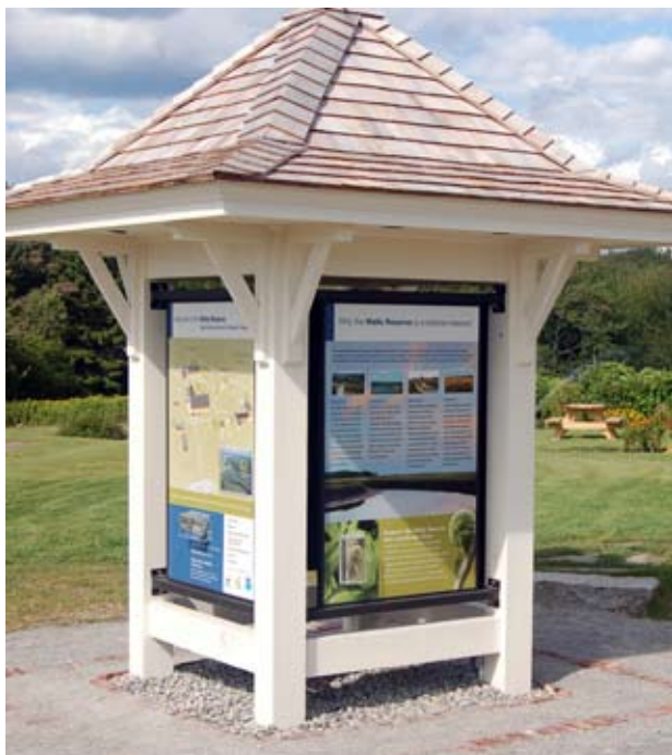
A new welcome kiosk was constructed in spring 2009.
