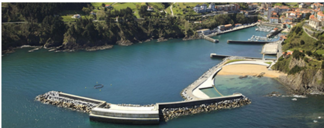
Figure 5.4. The Mutriku Wave Power Plant opened in July 2011 and provides harbor protection while generating electricity by harnessing air compressed by the action of waves, showing a positive benefit of MRE devices. The plan has 16 turbines with a total capacity of 296 kW (Ente Vasco de la Energía, http://www.eve.eus/Proyectos-energeticos/Proyectos/Energia-Marina.aspx?lang=en-GB ).
