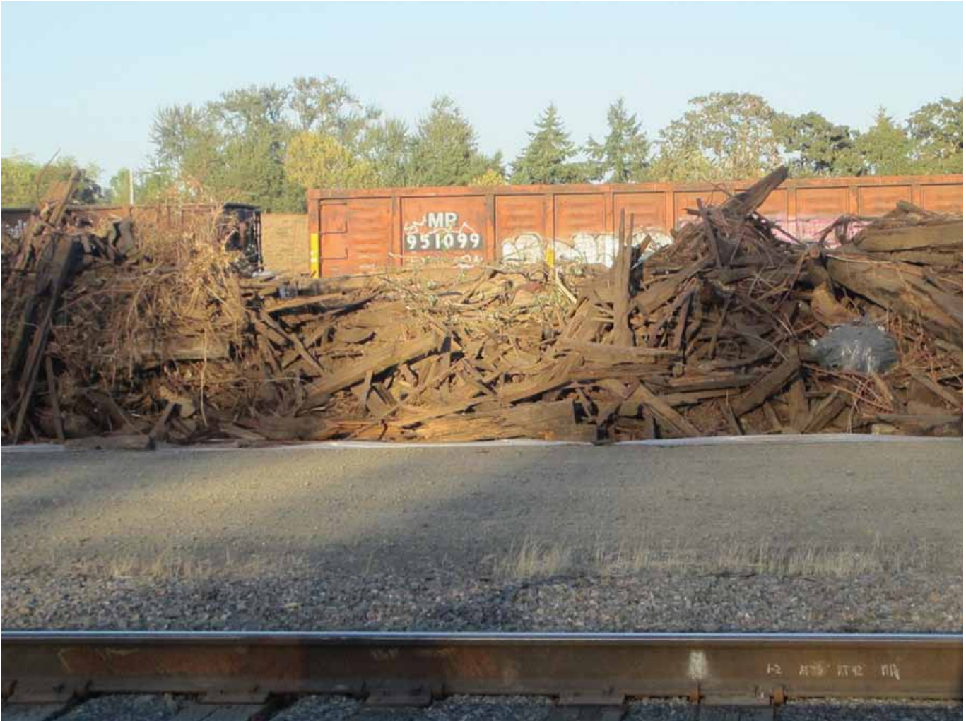
Creosote Logs pulled from Maxwell Pond during Hazardous Waste Clean Up (photo above and next page)
